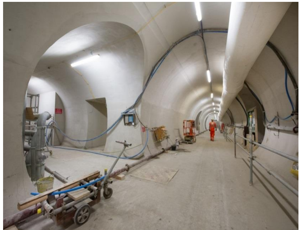
Central line passenger tunnel and overbridge
