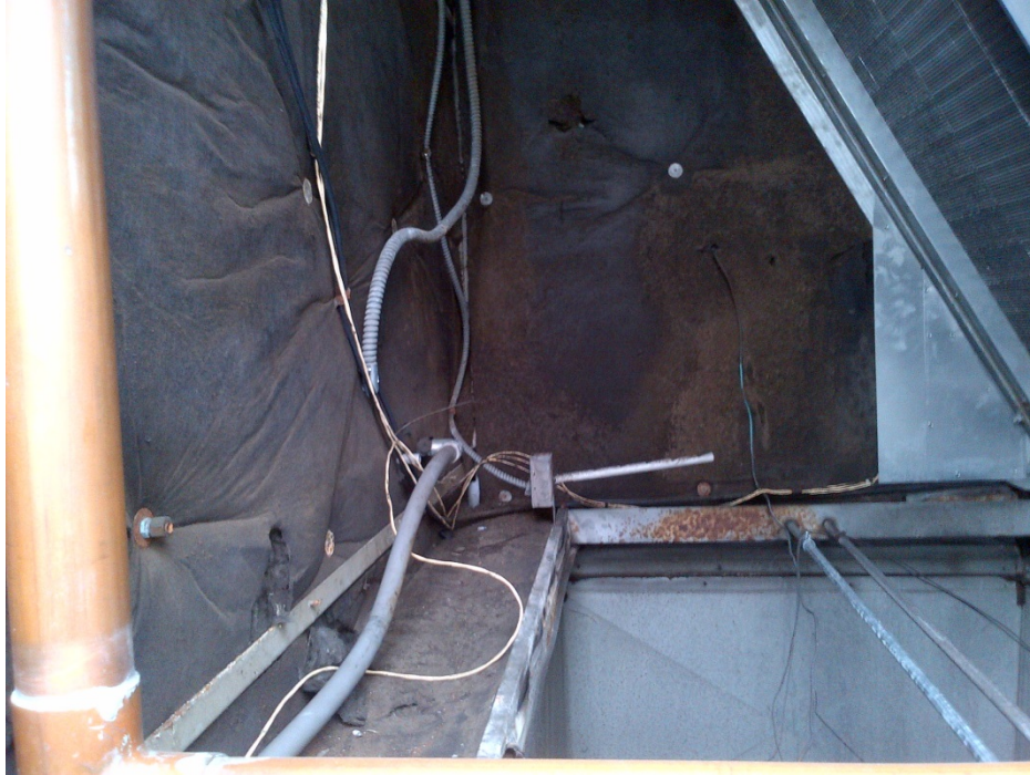
Insulation Liner in Air Handler Unit
