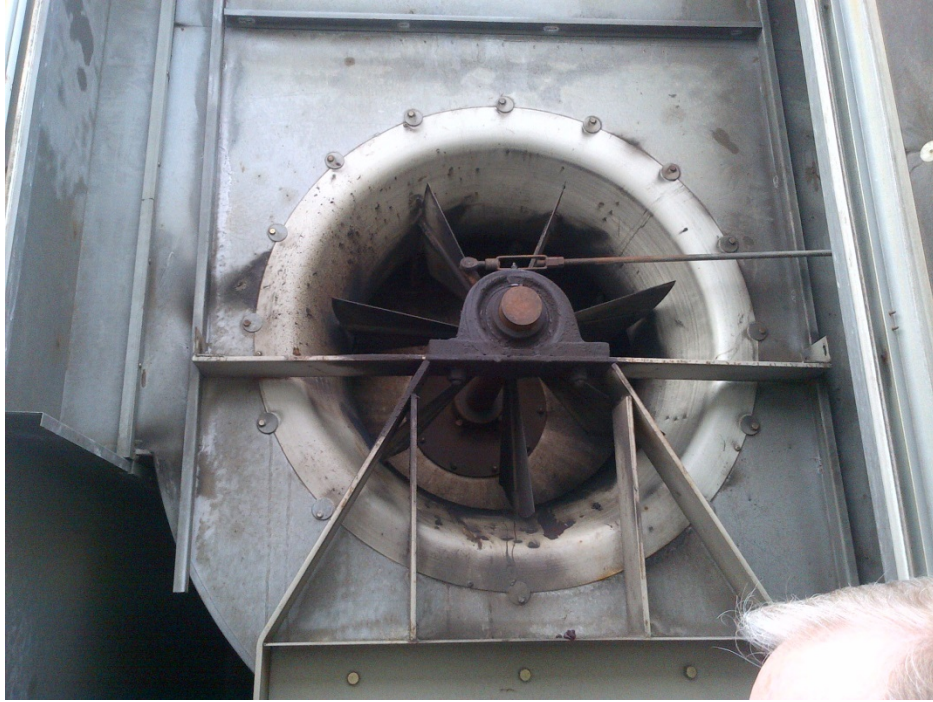
Interior of Air Handler Unit
