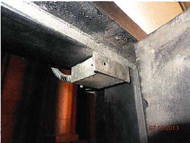
PIT DOOR CONTACT MISSING ACTIVATING BUTTON
