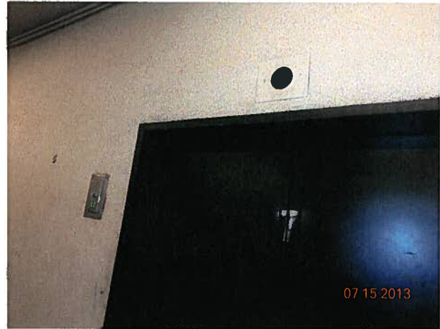
HALL LANTERN LENS MISSING CAR #7
