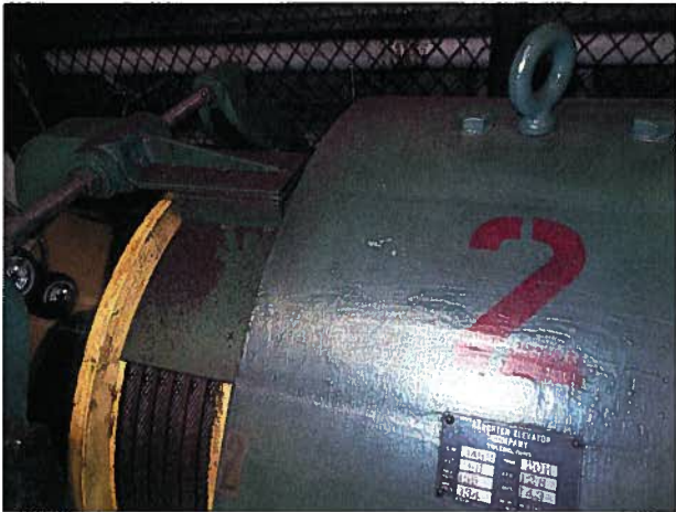
ROPE DUST ACCUMULATING ON MACHINE
