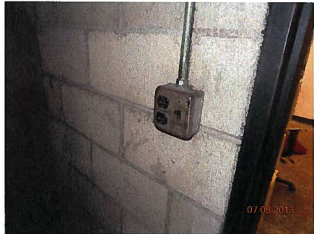
DUPLEX OUTLET IS NOT GFCI
