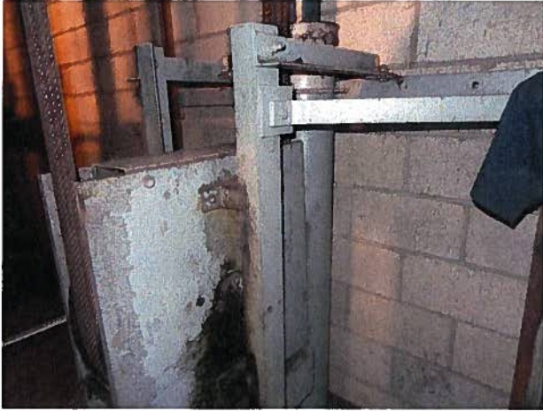
GREASE BUILD UP ON COMPENSATION SHEAVE
