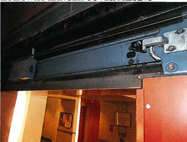
HOISTWAY HANGER COVER MISSING
