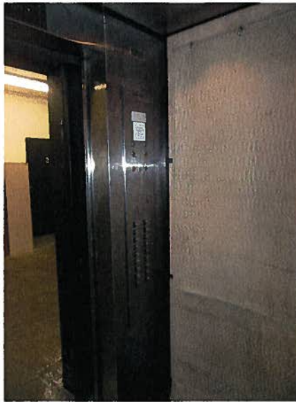
DOORS DO NOT OPEN THE FULL CLEAR WIDTH
