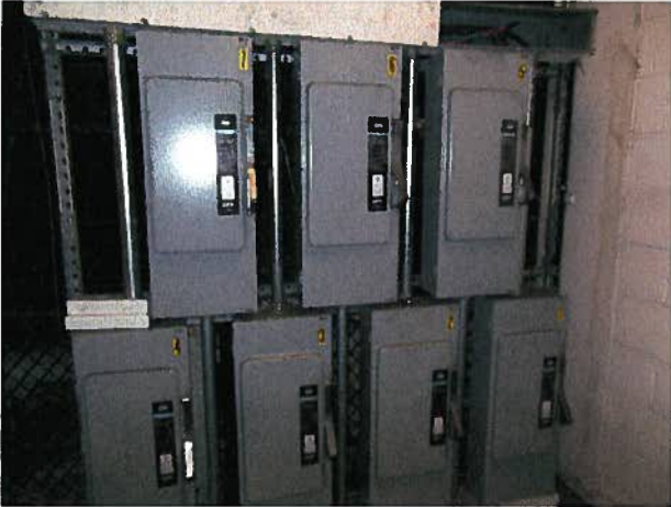
NO ELECTRICAL PANELS ID ON SWITCHES
