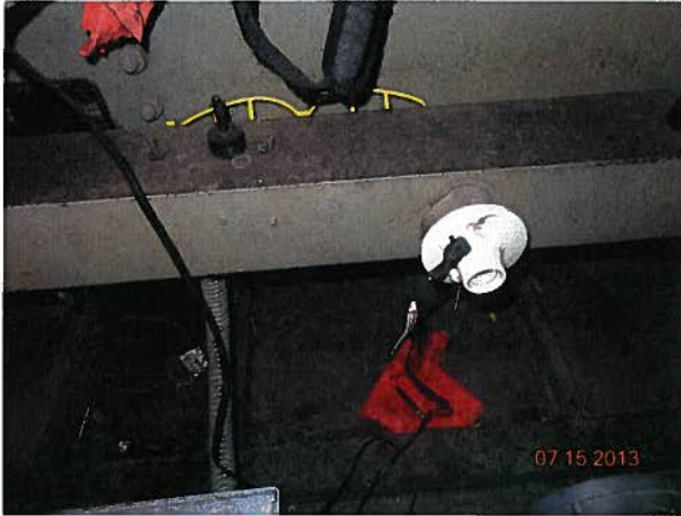
CAR TOP LIGHT MISSING BULB
