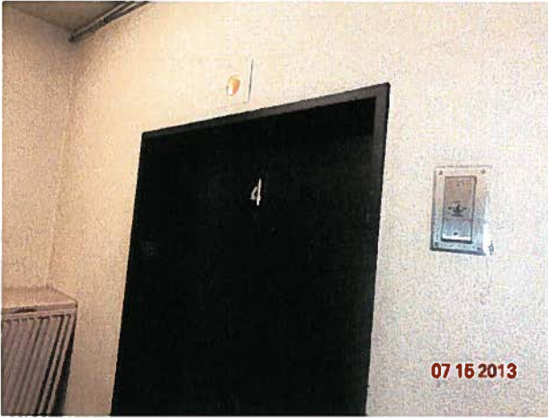
HALL LANTERN LENS MISSING CAR #4
