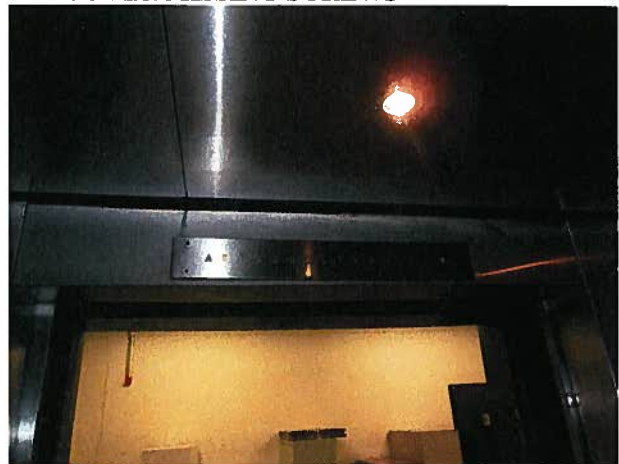
CPI COVER MISSING SCREWS
