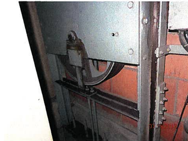
DIRT BUILD UP ON CWT. ASSEMBLY
