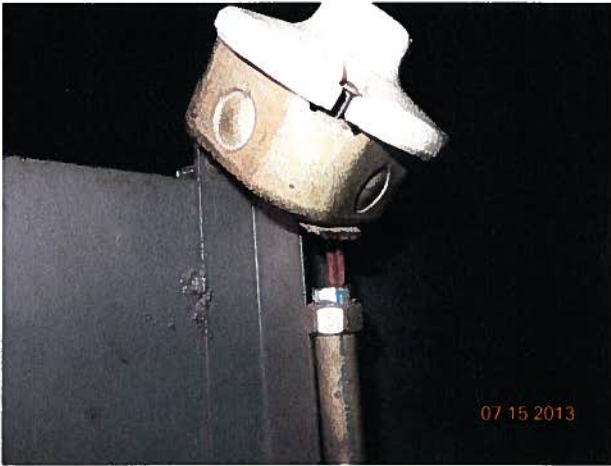
EXPOSED WIRES
