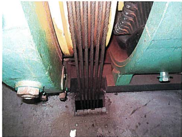
EVIDENCE OF ROPE AND SHEAVE ROUGE
