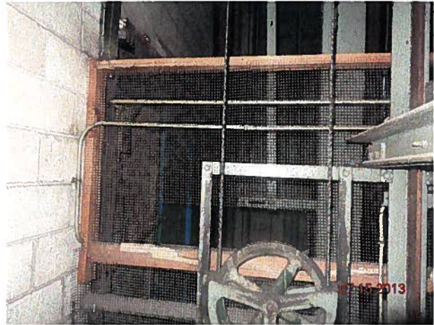
WOOD ENCLOSURE BETWEEN CARS #6 & #7
