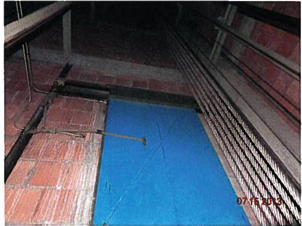
NO HOISTWAY FASCIA AT REAR OF CAR #7
