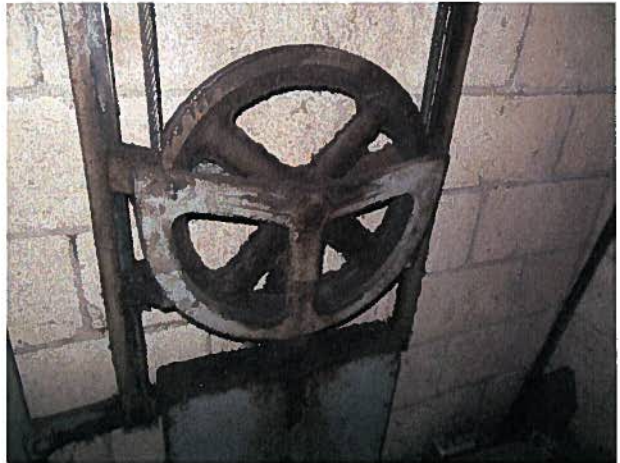
GOVERNOR TENSION SHEAVE DIRT BUILD UP
