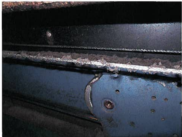
DIRT BUILD UP ON CAR DOOR HANGER
