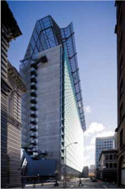
Figure 2. Type 316 perforated screens on the San Francisco Federal Building helped eliminate air-conditioning in 70% of the building's occupied spaces. © Iwan Baan Studio
