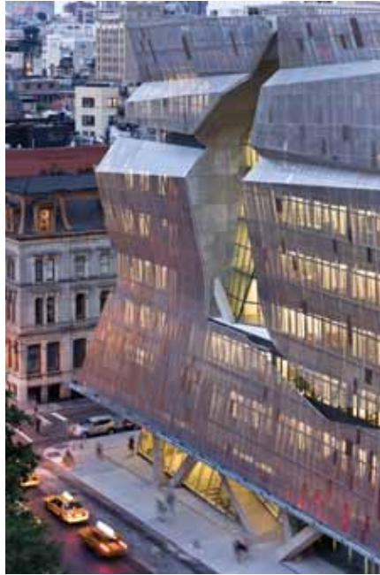
Figure 3. Perforated Type 304 screens give 41 Cooper Square a sculptural appearance while reducing the building's energy consumption. © Iwan Baan Studio
