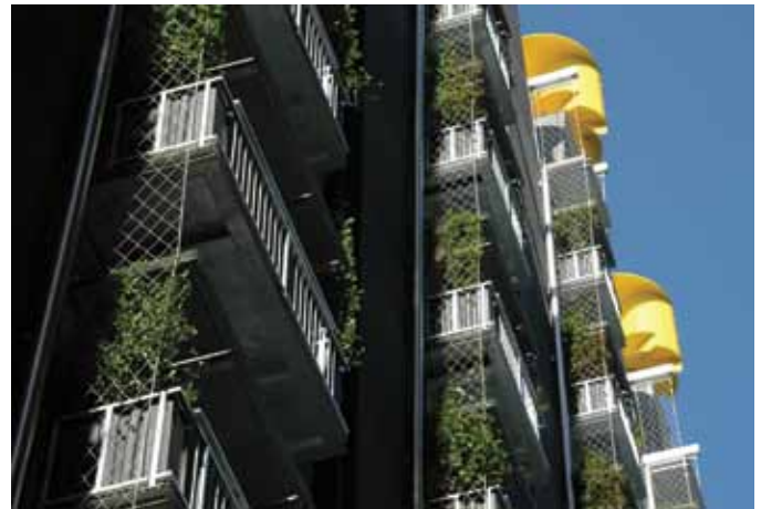
Figure 8. Plant screens were used along the balconies on the north side of Council House No. 2 and over the roof deck to shelter them from sun. © Ronstan Tensile Architecture
