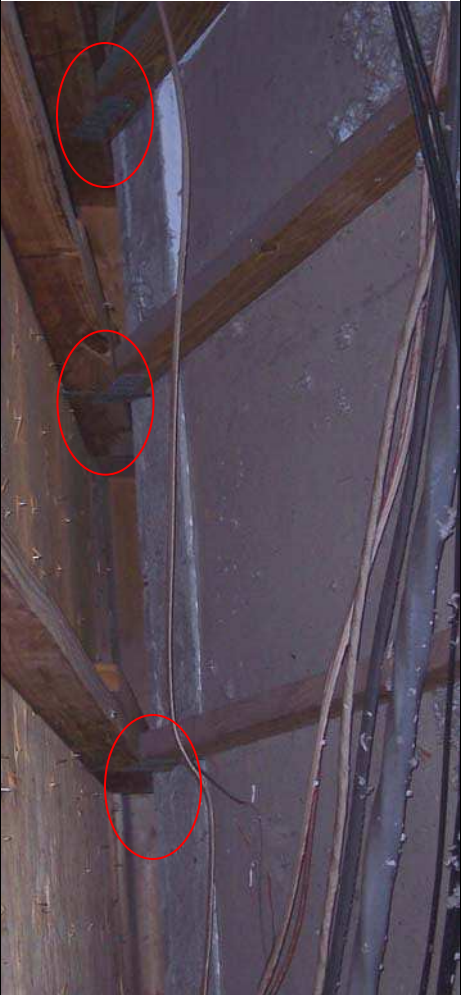
Single Wrap Tie-Down Straps on each truss
