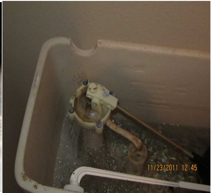
PHOTO NO. 20 COMMODE TANK MISSING ANTI-SIPHONING DEVICE
