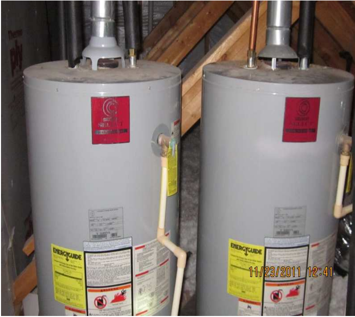
PHOTO NO. 19 WATER HEATER PIPING CONNECTIONS MISSING DIELECTRIC FITTINGS
