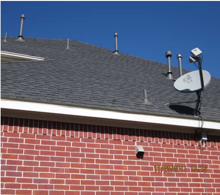
PHOTO NO. 27 TURNED UP ROOF SHINGLES ON SOUTH SIDE ROOF
