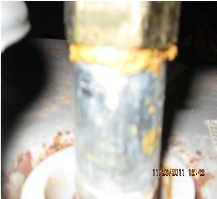
PHOTO NO. 19 WATER HEATER PIPING CONNECTIONS MISSING DIELECTRIC FITTINGS
