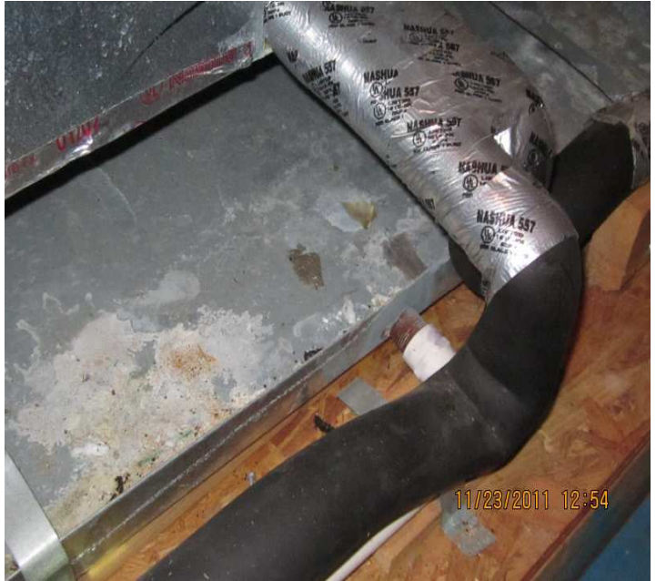
PHOTO NO. 24 A/C DRAIN PAN, IN ATTIC, MISSING FLOAT SWITCH
