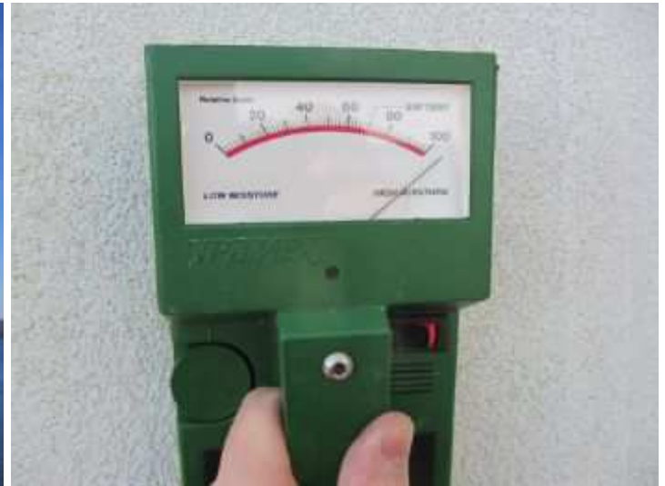
Tramex wet wall detector reading 100%
