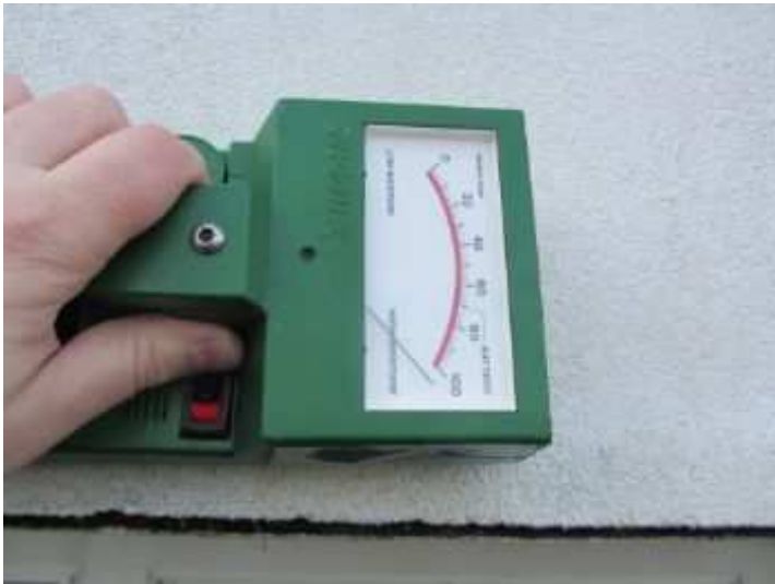
Tramex wet wall detector reading 100%
