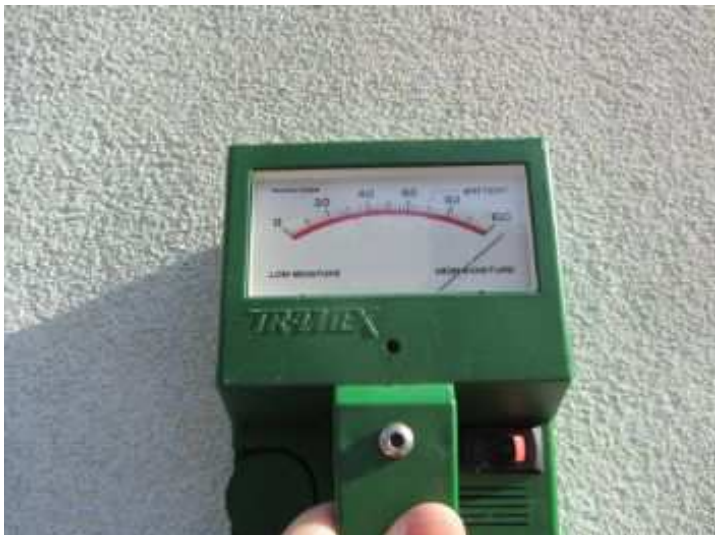
Tramex wet wall detector reading 100%
