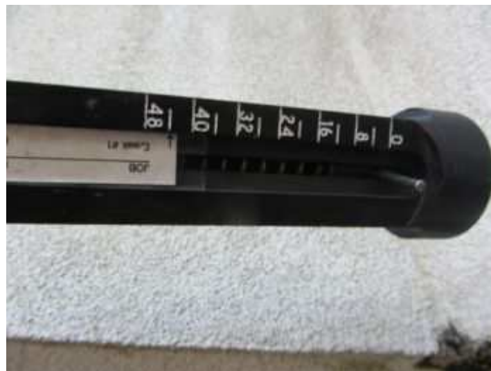
Tests with the Structure Resistance Tester (SRT) was 48 pounds of resistance without any penetration into the wood.
