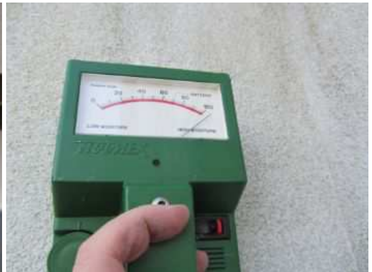
Tramex wet wall detector reading 100%
