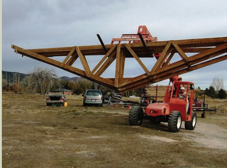
Roof joists are removed from a building to be transferred to ReSource in Boulder.
