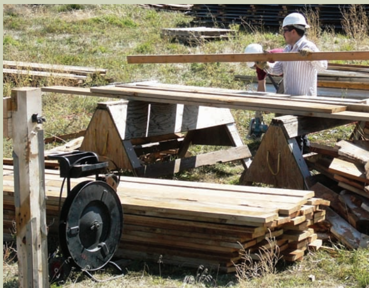
Deconstruction saves lumber from the landfill and prepares it for reuse.
