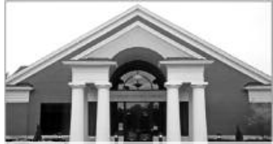
Servicing the residents of Woodhaven.
