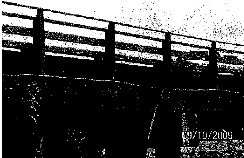
Steel Rail Post Attachment
