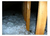
STRUCTURE Roof structure material is wood, Truss framing, Sheathing material is flakeboard.
