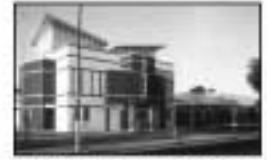
West Contra Costa USD Bond Program, $458 Million Program and Construction Management
