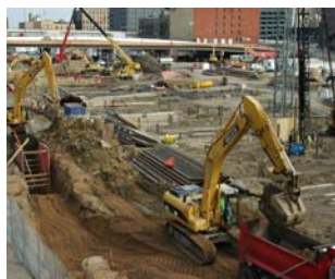
Double Stack Trench-Box
