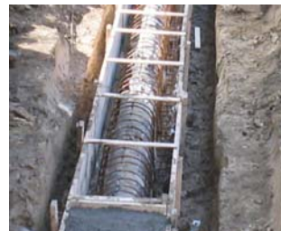
Concrete Encased Watermain
