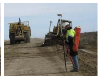
In-house GPS Survey
