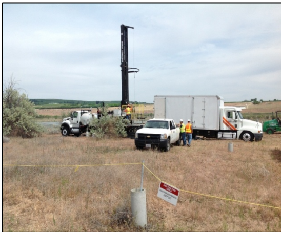
Deep (200 - 250 Ft) Borehole Drilling Near Columbia River (Hanford and Pasco) for Natural Gas Pipeline Environmental Impact Statement.
