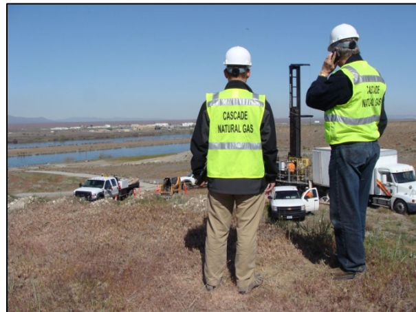
Deep (200 - 250 Ft) Borehole Drilling Near Columbia River (Hanford and Pasco) for Natural Gas Pipeline Environmental Impact Statement.
