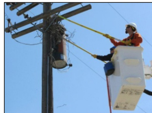
Removing a bird's nest from a power pole
