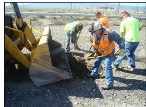
Teamsters & Heavy Equipment Operators hand-dig the oil spill
