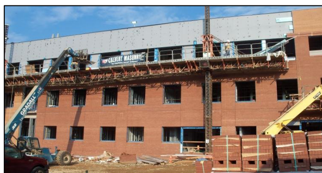
Figure 10 - View looking at east elevation. Fraco Lifts are used around exterior to provide efficient flow of construction along a large percentage of elevation at a time. Materials are lifted into place with a boom lift. Personal photograph taken by Chris Pozza.
