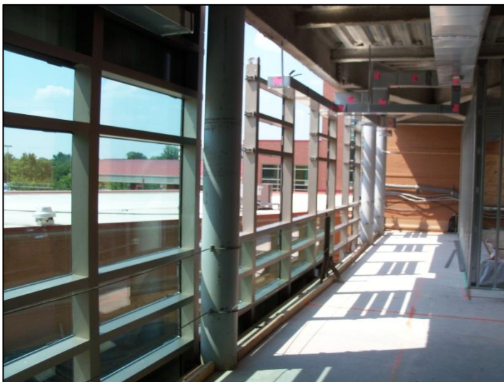
Figure 12, left – Interior view of west elevation curtain wall system under construction. Personal photograph taken by Chris Pozza.
