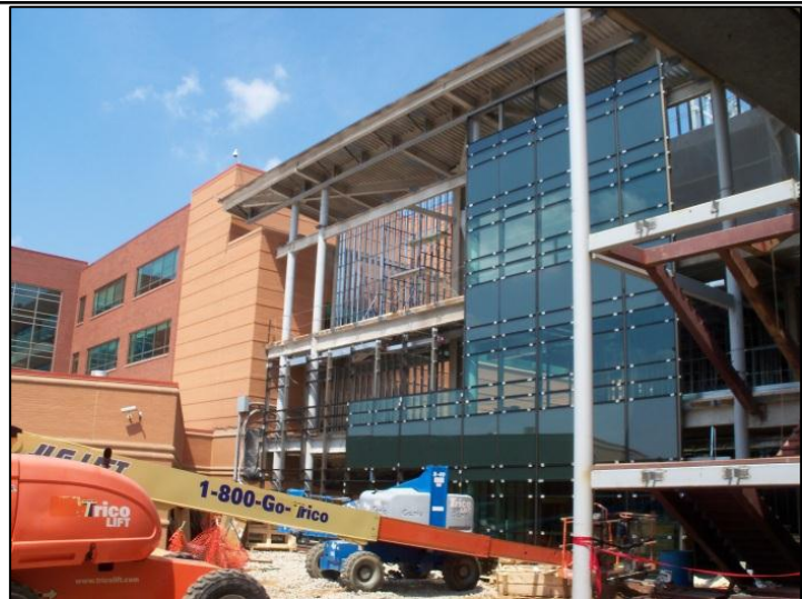
Figure 11 - View of west elevation curtain wall system under construction. The boom lift used during construction of the façade system can be seen at the bottom of the photo. Personal photograph taken by Chris Pozza.
