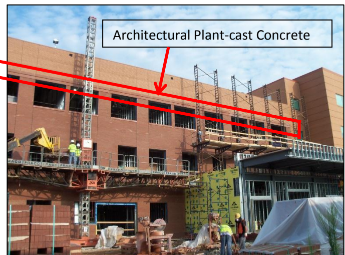
Figure 1, Below - Architectural precast concrete is seen under window sills and spanning the addition on the left above the third story windows. Personal Photograph taken by Chris Pozza.
