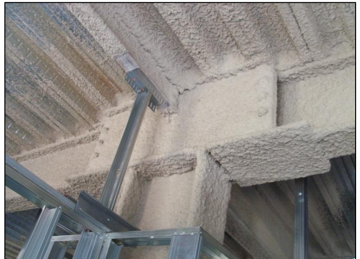
Figure 2 – Photograph of a Sideplate system. This is a moment frame that connects columns to beams and girders and can be single or double sided, shown above is a double-sided connection. Spray-on fireproofing has already been applied to the structural steel at this point of construction. Personal photograph taken by Chris Pozza.
