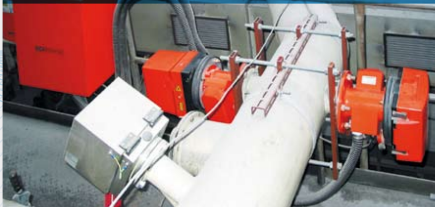
Hydrogen fluoride measurement in a hospital waste incinerating plant
