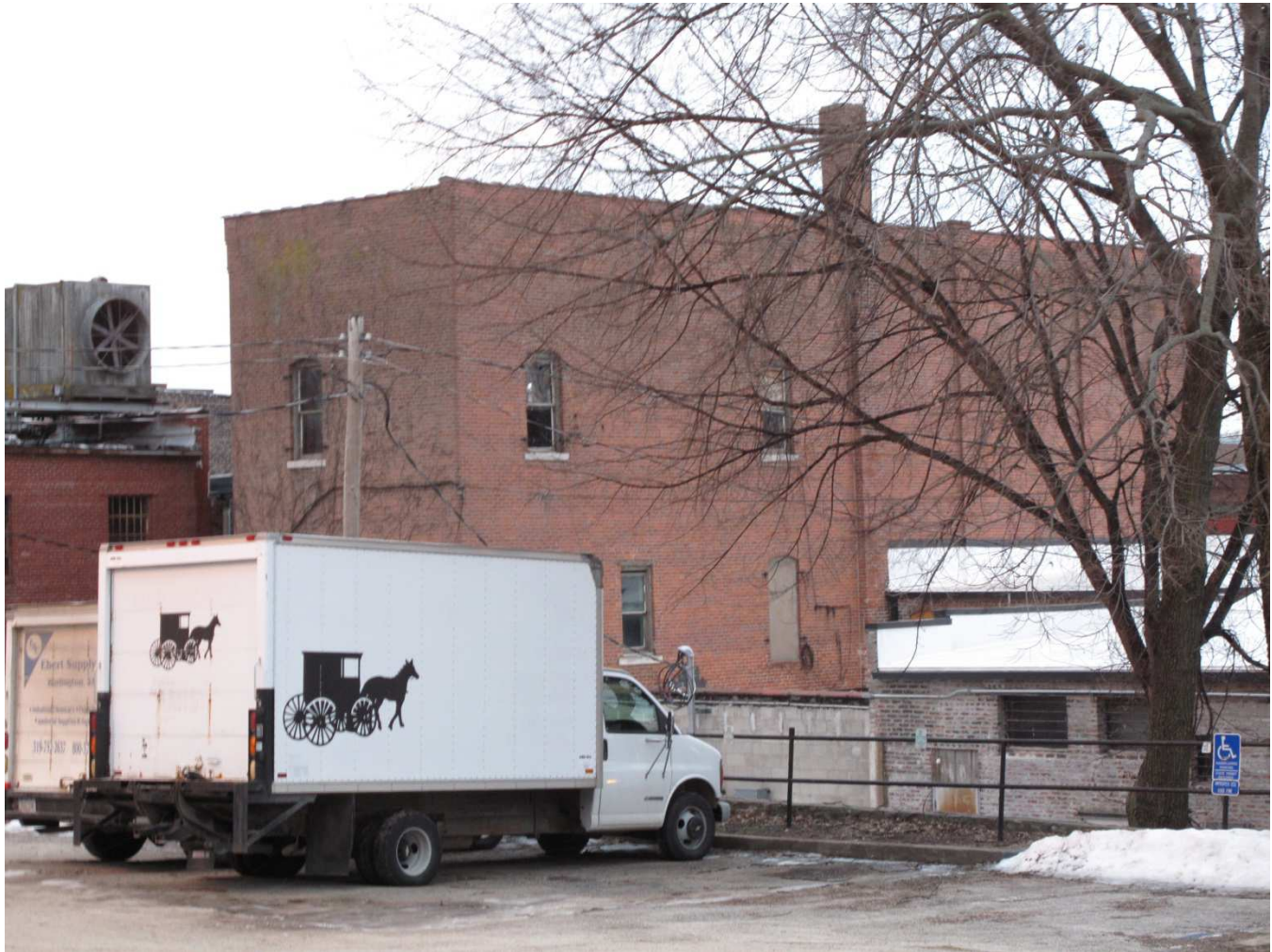
Photograph 29-01114-003 – North and west elevations, looking southeast (McCarley, January 14, 2014).
