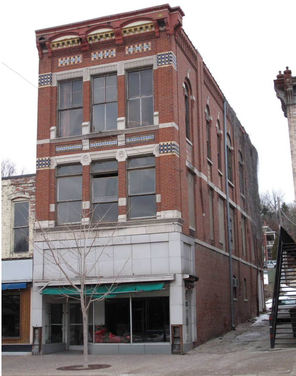
Photograph 29-01114-001 – South and east elevations, looking northwest (McCarley, January 14, 2014).
