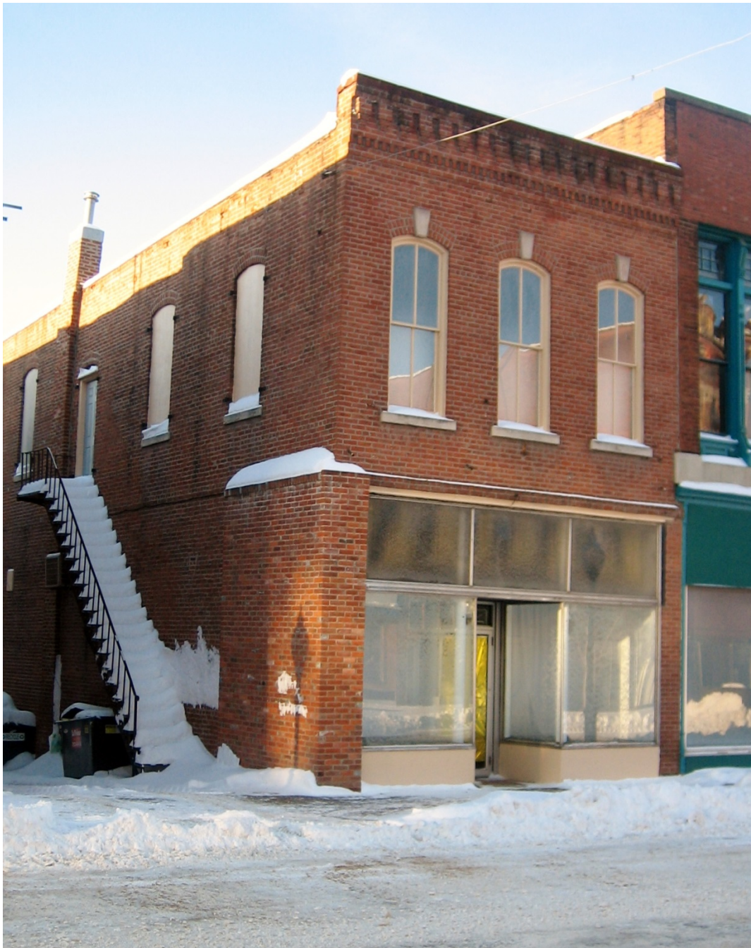
Photograph 29-01115-001 – East and north elevations, looking southwest (Frevort, February 6, 2013).
