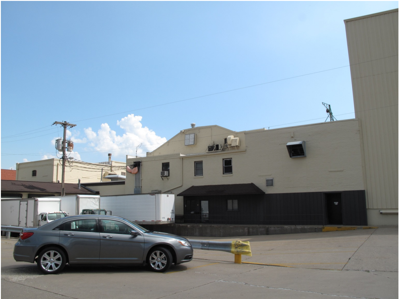
Photograph 29-03094-002 – North elevation, looking south (McCarley, July 17, 2013).
