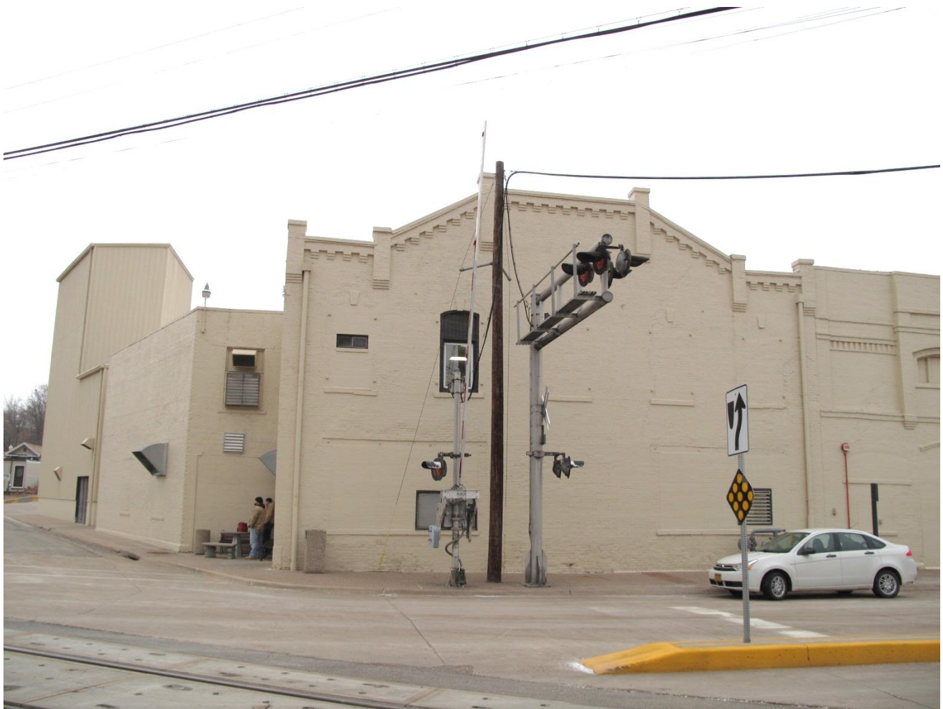
Photograph 29-03094-001 – South elevation, looking north (McCarley, January 14, 2014).
