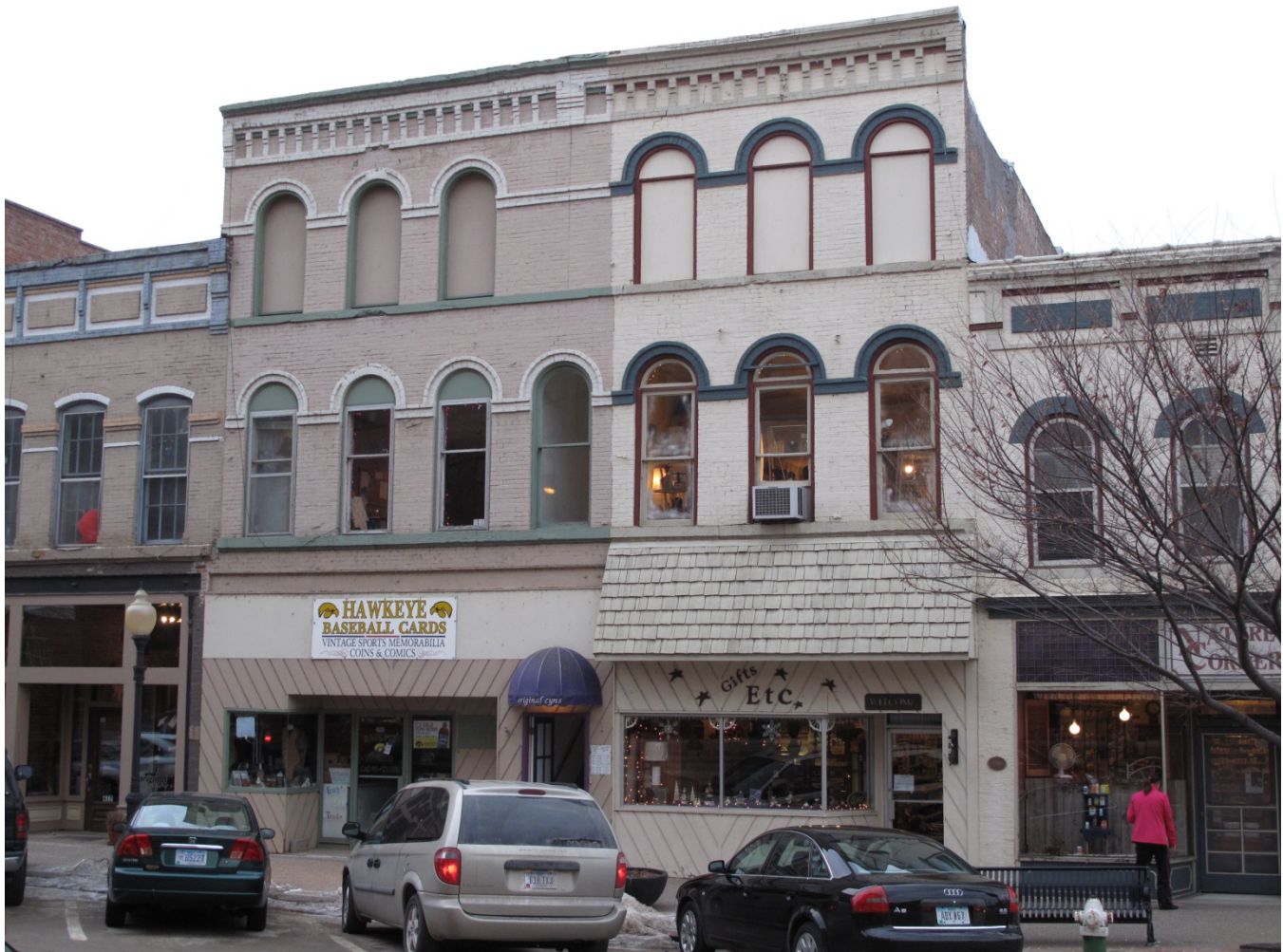
Photograph 29-01105-001 – North elevation, looking south (McCarley, January 14, 2014).
