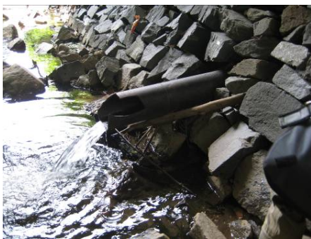
An outfall discharging during dry weather
