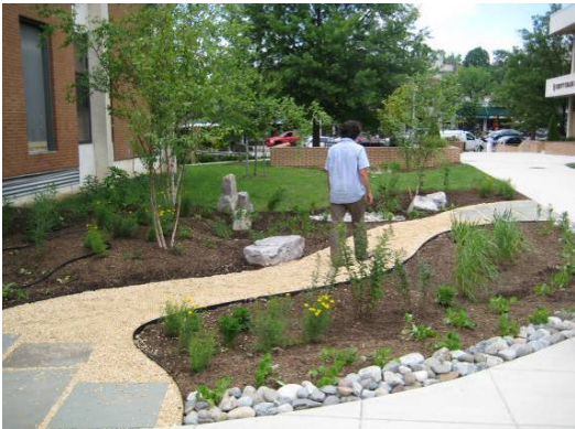
A rain garden demonstration site at a recreation center
