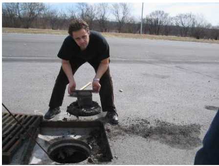
A catch basin insert with collected pollutants
