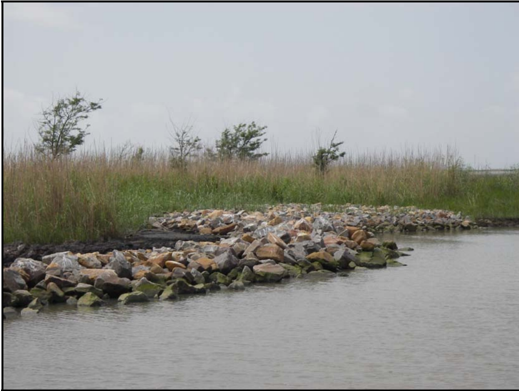
Photo No. 7, Closure No. 3 bank paving west side
