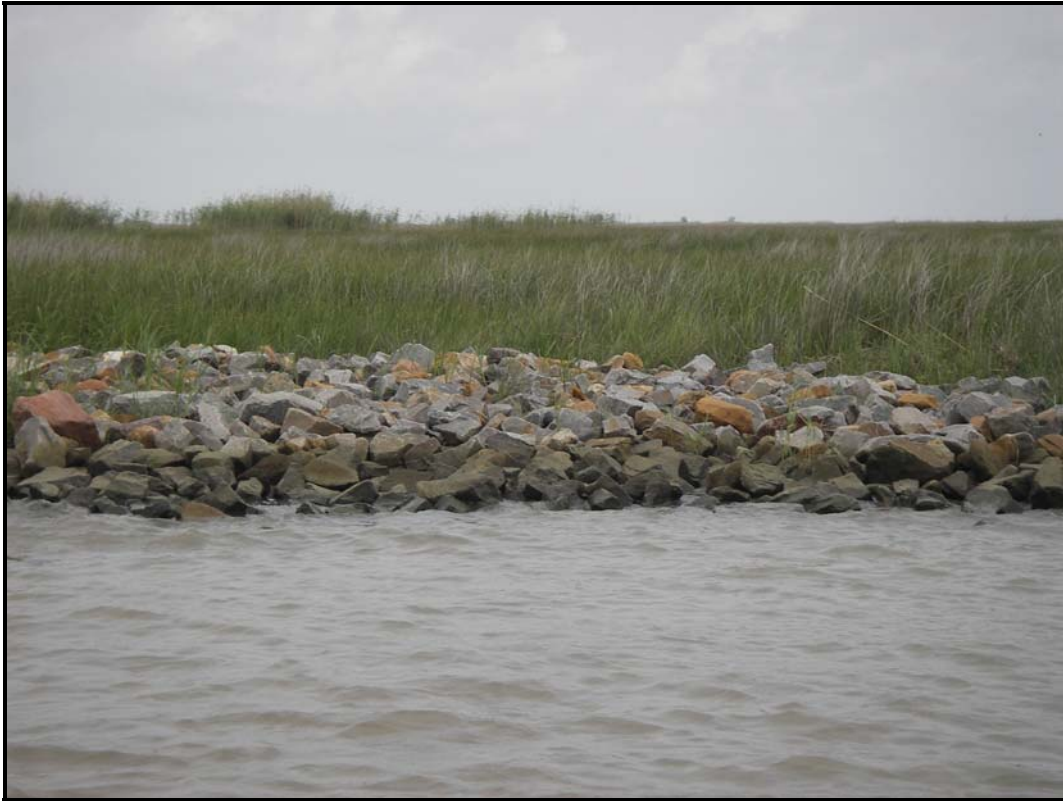
Photo No. 15, Closure No. 6 bank paving north side
