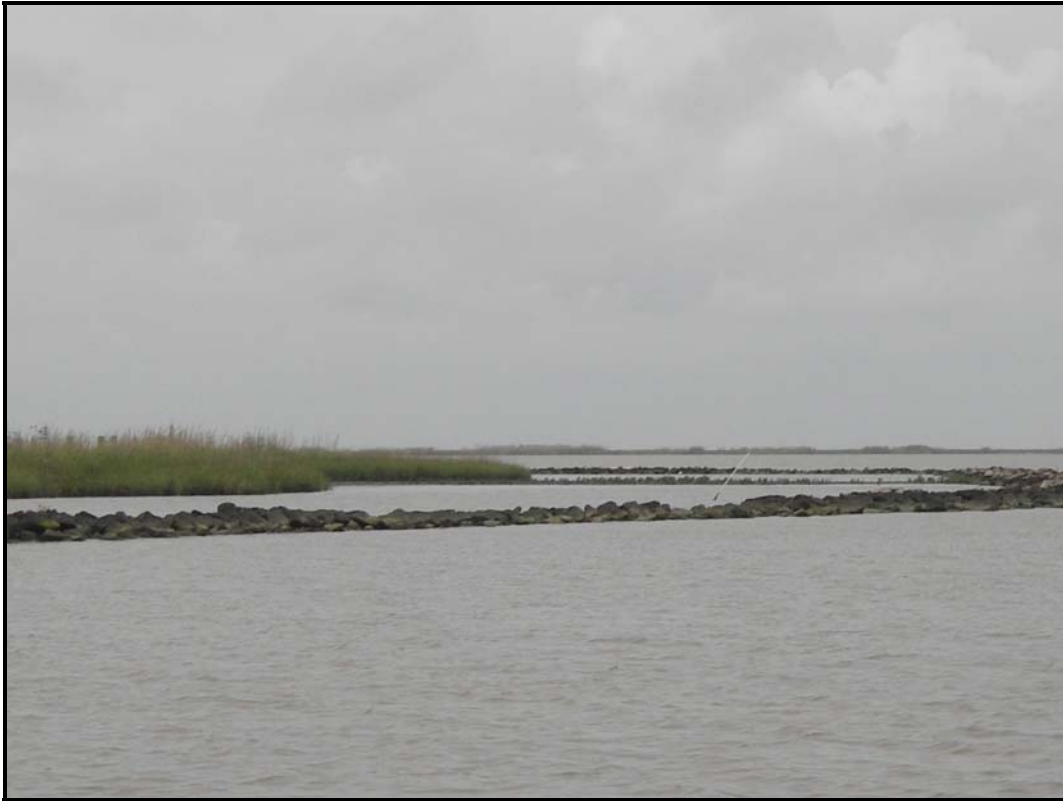
Photo No. 17, Structure No. 7 marsh creation behind rock dike starting to vegetate
