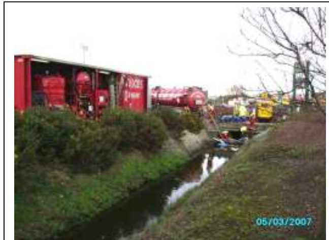
Tyock Burn culvert cleaning
