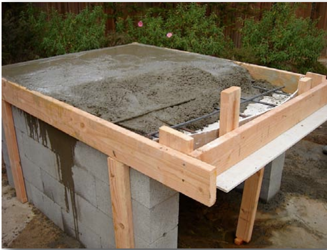
4.1. Rebar set in center of the concrete pad.
