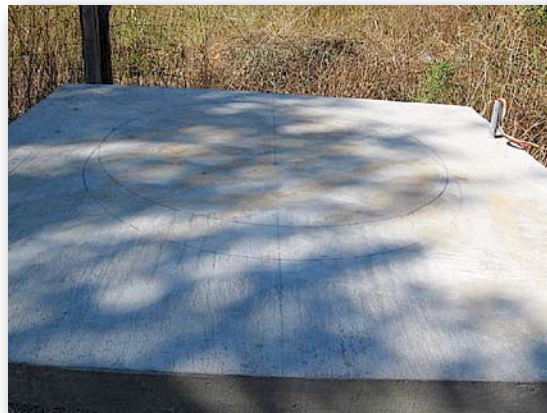
5.3 Measure carefully where the oven will sit.
