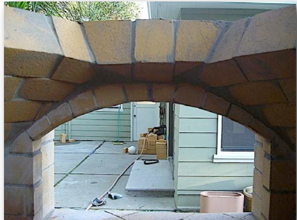
8.3. The intersection between the dome and opening.
