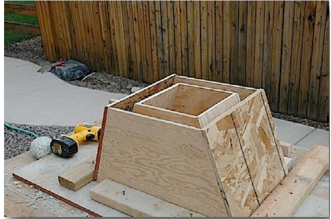
10.5. Construct the form using plywood.
