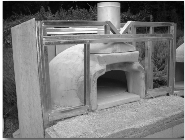
16.5 Metal studs walls with a shed roof.
