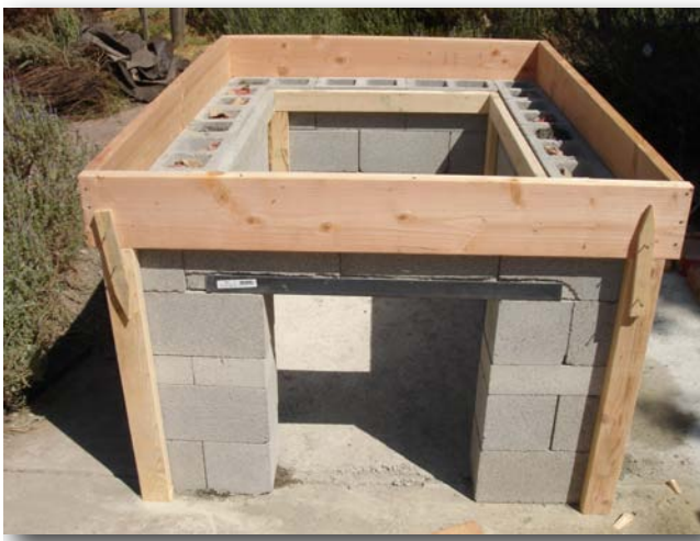
3.5 Form sides held in place with 2"x4"s.
