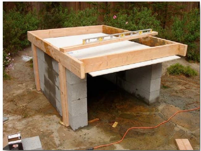
3.3. Hardibacker inside the side forms.
