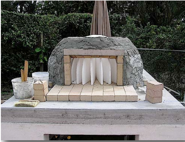
8.5. A cast lintel forms oven opening.
