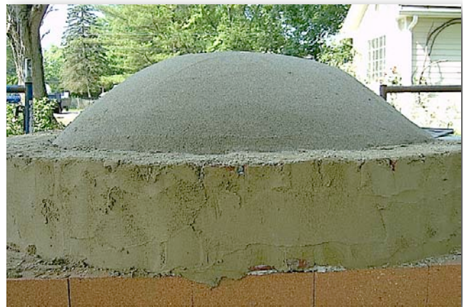
6.4 Sand form inside first course for bricks.
