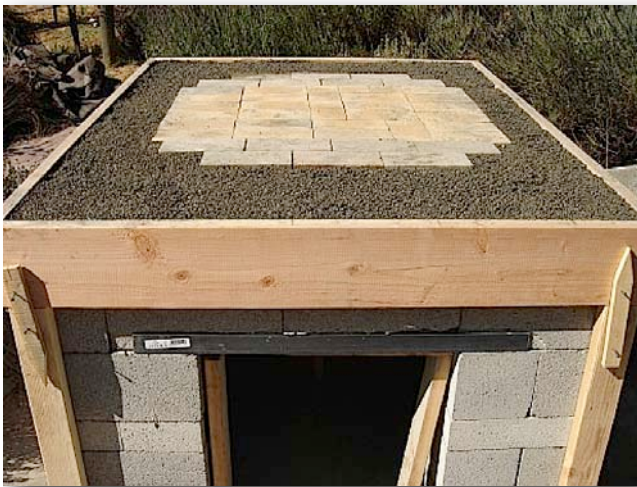
3.7. Firebrick splits under the cooking floor.
