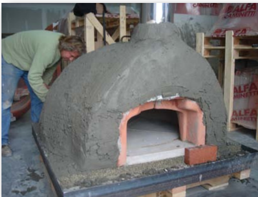
15.5 Rough coat of stucco on wire lathe.
