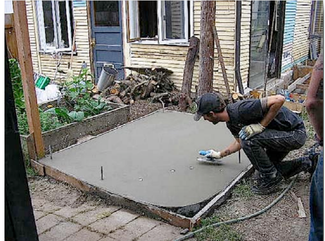
1.5 The finished foundation ready to cure.
