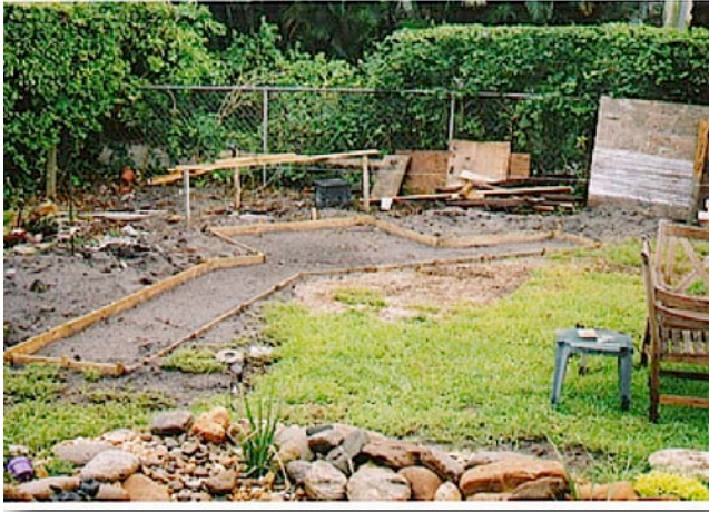
1.6. A complete outdoor kitchen foundation.
