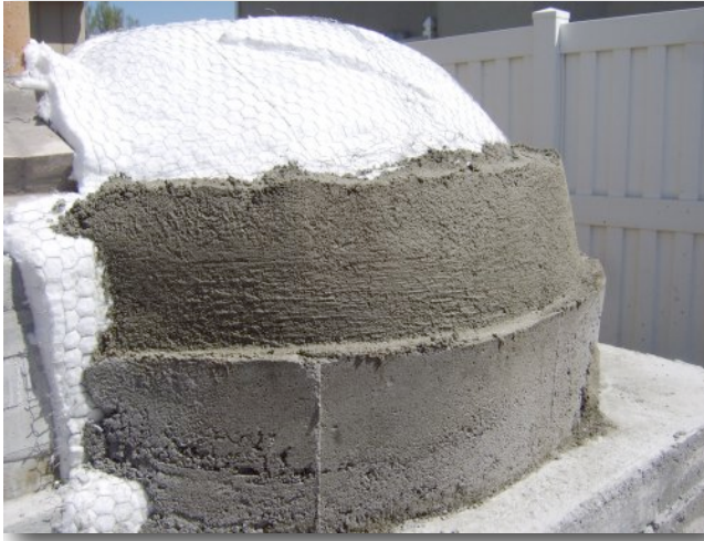
13.3 FB Blanket covered with wire and insulating concrete.
