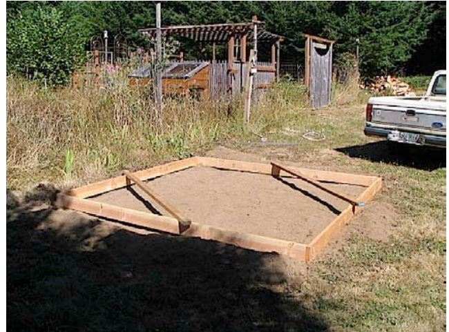
1.8. 2"x4"s hold the form square and plumb.
