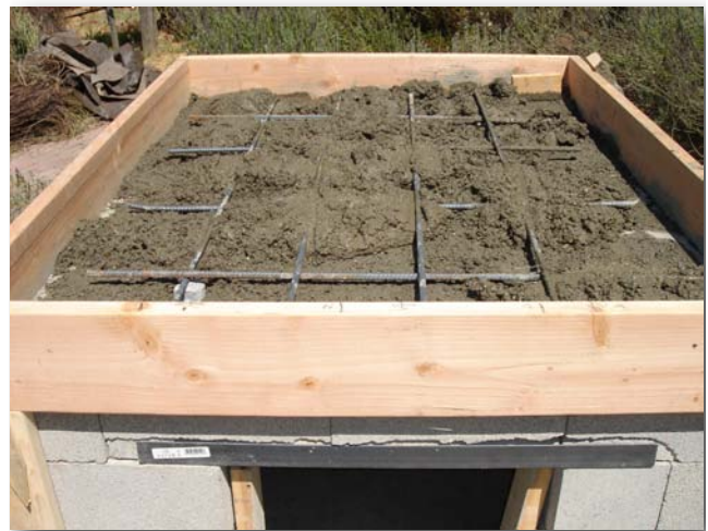
4.3. Rebar set in center of the concrete pad.
