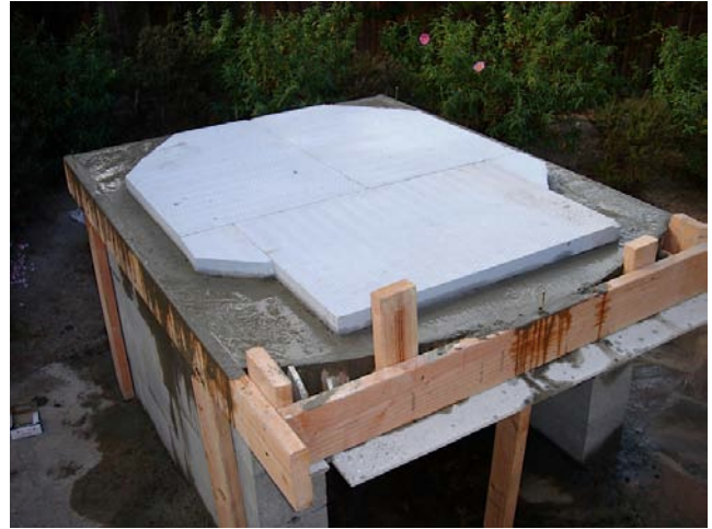
4.2. FB Board on damp concrete.
