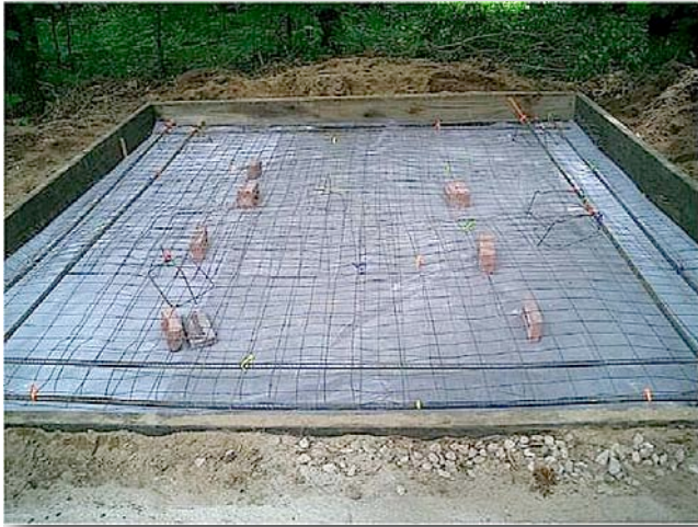
1.3. Framed, lined, with wire mesh and rebar.
