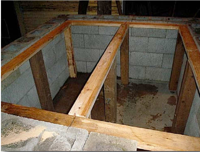
3.1. The form support ready for the tray.
