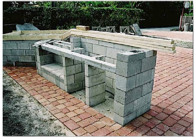
2.2. Stand with cast lintels.
