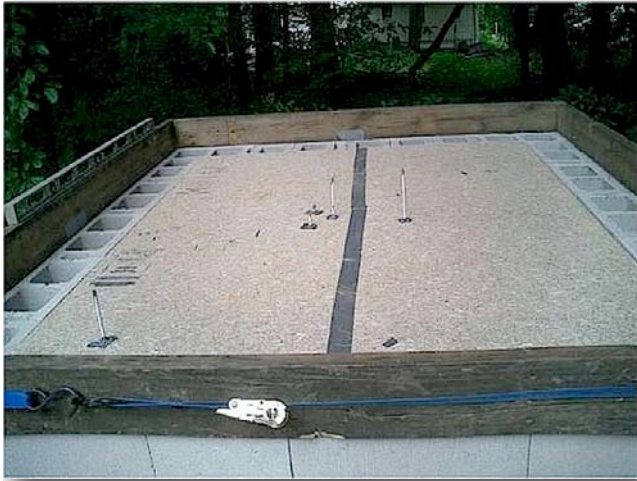
3.4. Plywood set in place.
