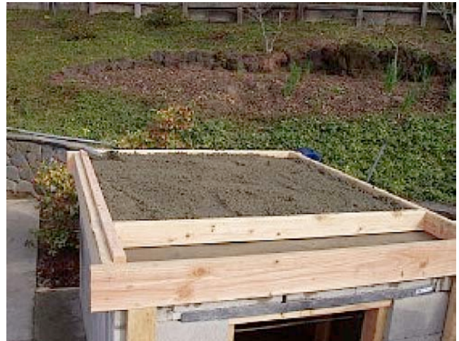
4.6. Vermiculite concrete poured under the oven chamber.
