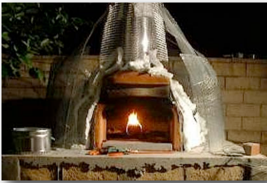
15.4 Rebar and lathe shape the Igloo.
