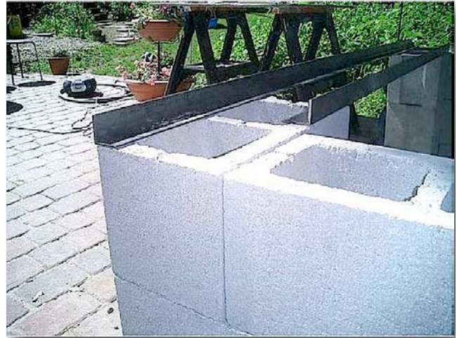
2.5. Cut the back angle iron to leave room for blocks.
