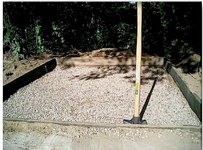
1.2. A gravel or crushed rock bed.
