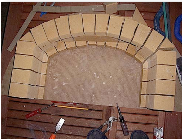
8.6. The entry arch and vent has a clearly defined door stop.
