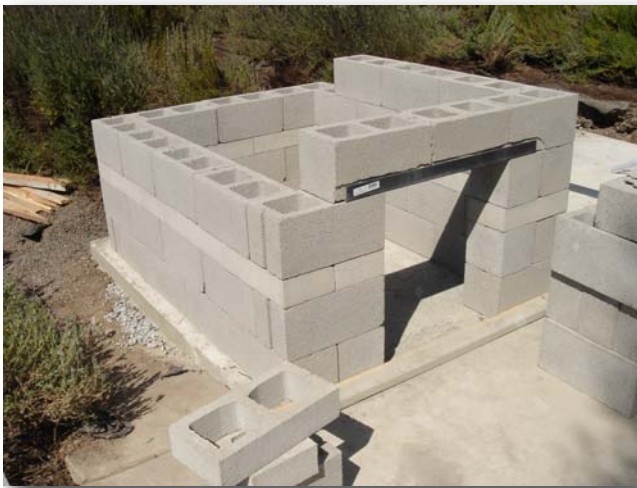
2.1 Angle iron supports the fourth block course.
