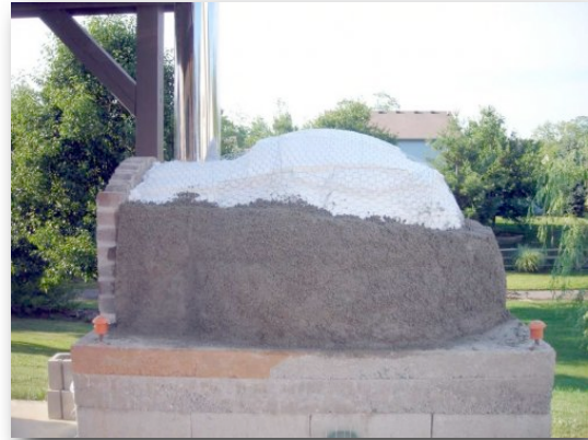
15.6 The Igloo shape coming together.
