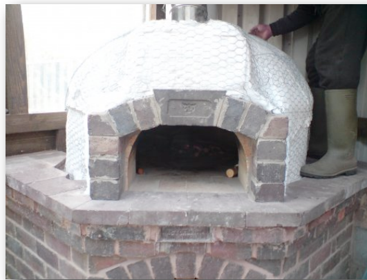
13.2 Multiple layers of FB Blanket.
