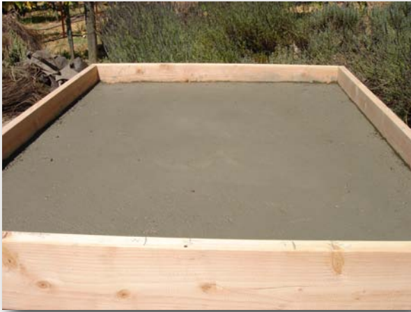
4.4. Structural layer waiting on insulating layer.
