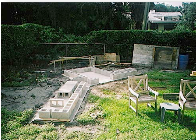
1.7 The foundation and first course of stand blocks.
