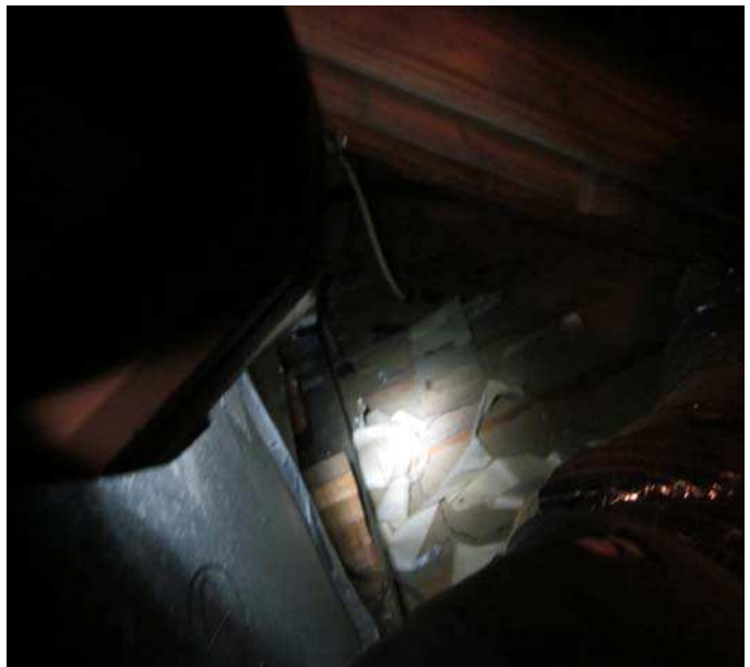
PHOTO NO. 20 A/C DRAIN PAN MISSING FLOAT SWITCH
