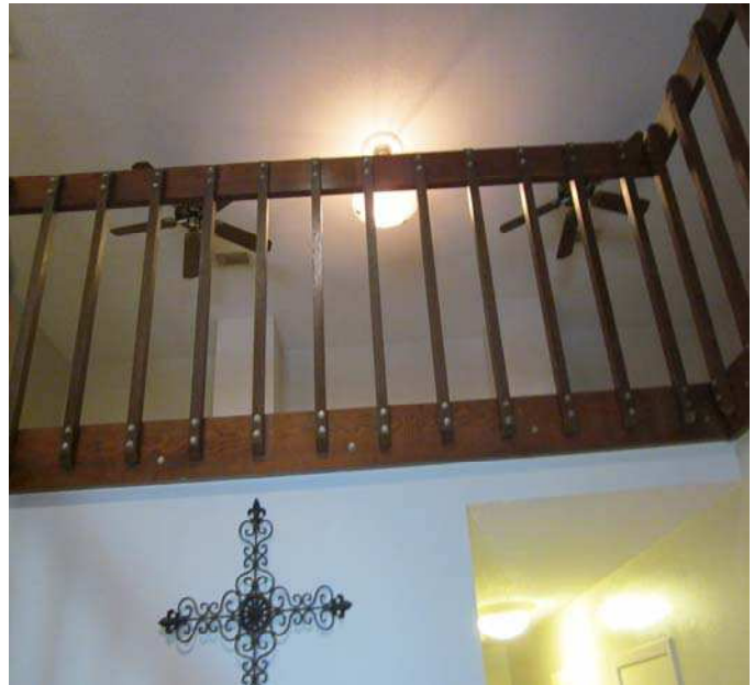
PHOTO NO. 16 GUARD RAIL SEPARATION DOES NOT MEET "4-INCH" RULE
