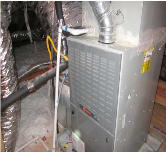
PHOTO NO. 23 VERTICAL A/C -FURNACE UNIT IN UPPER ATTIC
