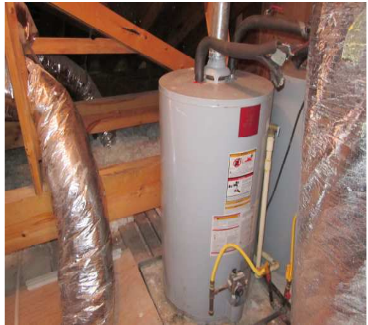
PHOTO NO. 24 TWO GAS WATER HEATERS IN LOWER BACK ATTIC
