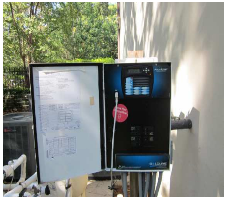
POOL PUMPING EQUIPMENT CONTROL BOX
