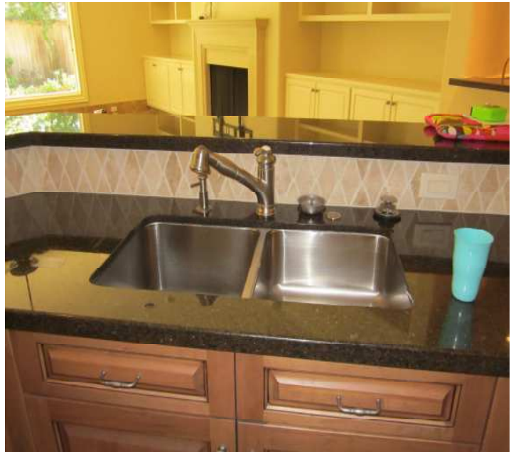
PHOTO NO. 16 KITCHEN SINK MISSING ANTI-SIPHONING DEVICE
