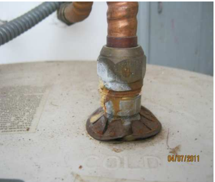
PHOTO NO. 4 CORRODED PIPING CONNECTION AT TOP OF WATER HEATER
