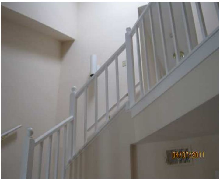
PHOTO NO. 8 STAIR GUARD RAIL DOES NOT MEET "4-INCH" RULE
