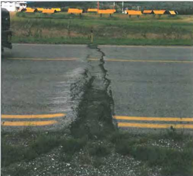
Photo 3: Taxiway B, Utility Jacking
