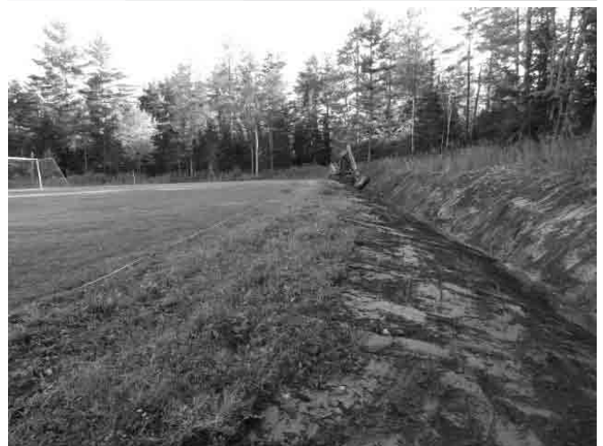
Drainage improvement project at the rec fields.
