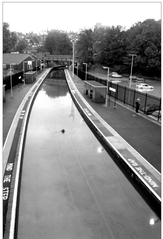
Fig. 8. The impact of the 2007 floods on rail infrastructure
