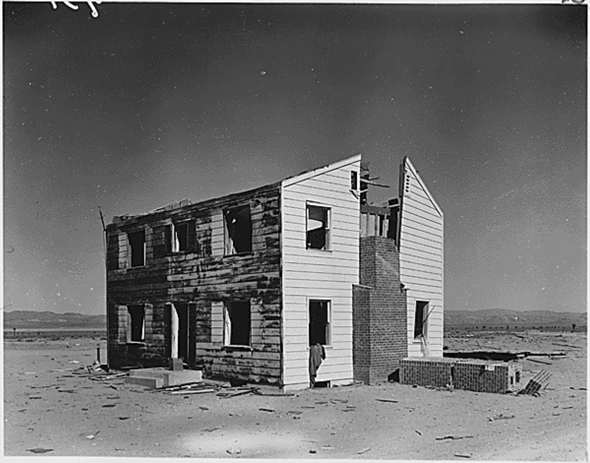
Photograph [Operation Cue] - Two-story wood frame house at 5,500 feet after the blast, May 5, 1955. ARC Identifier: 541788
