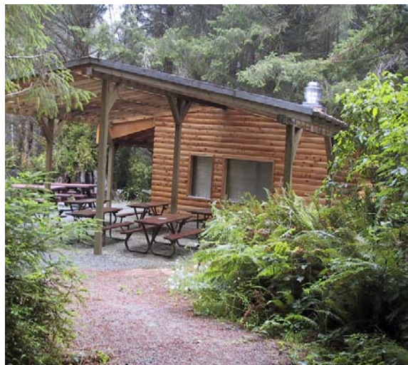
Kitchen and covered eating/classroom area
