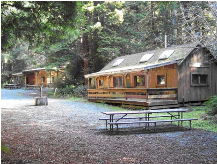
The old Lodge, with new kitchen area in the background
