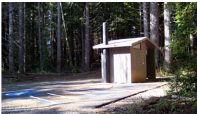
The composting toilet in parking lot
