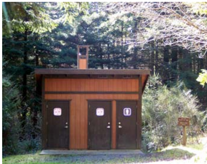
Clivus Multrum toilets, front view
