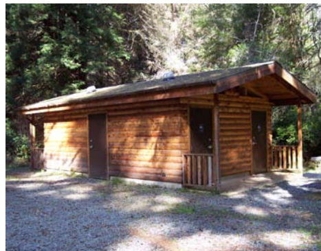
Restrooms, built in 2000
