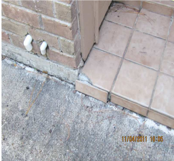
PHOTO NO. 12 DAMAGED TILE FLOORING ON WEST SIDE PORCH
