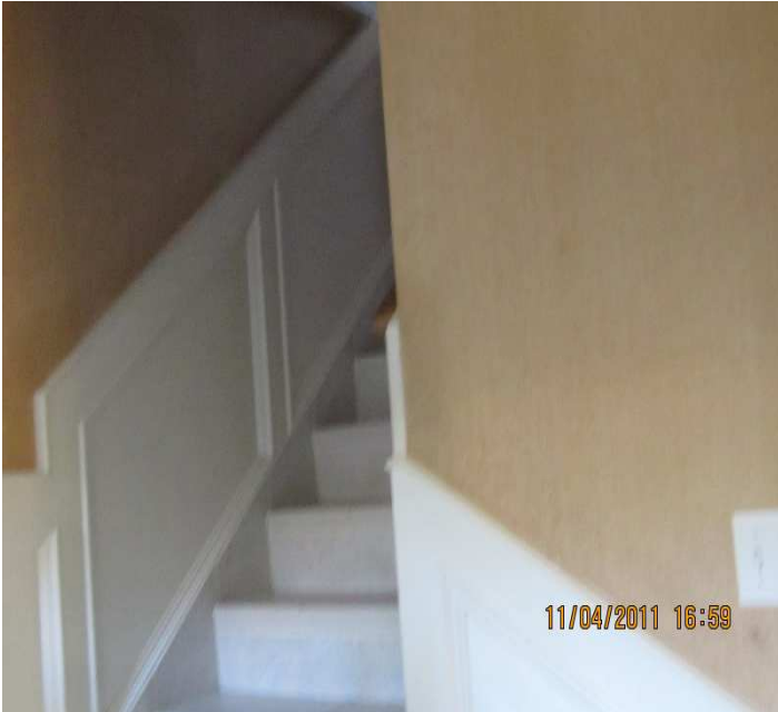
PHOTO NO. 23 STAIRWAY MISSING CONTINUOUS HAND RAIL
