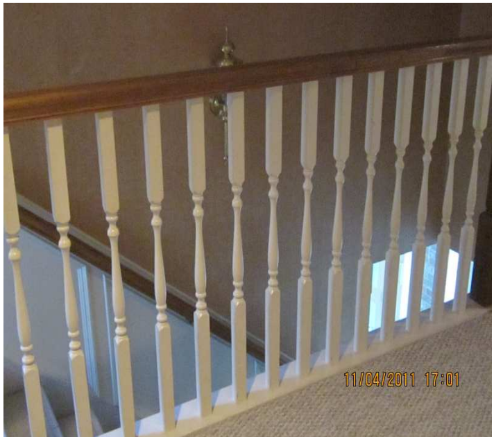
PHOTO NO. 24 GUARD RAIL, IN UPSTAIRS GAME ROOM, DOES NOT MEET "4-INCH" RULE
