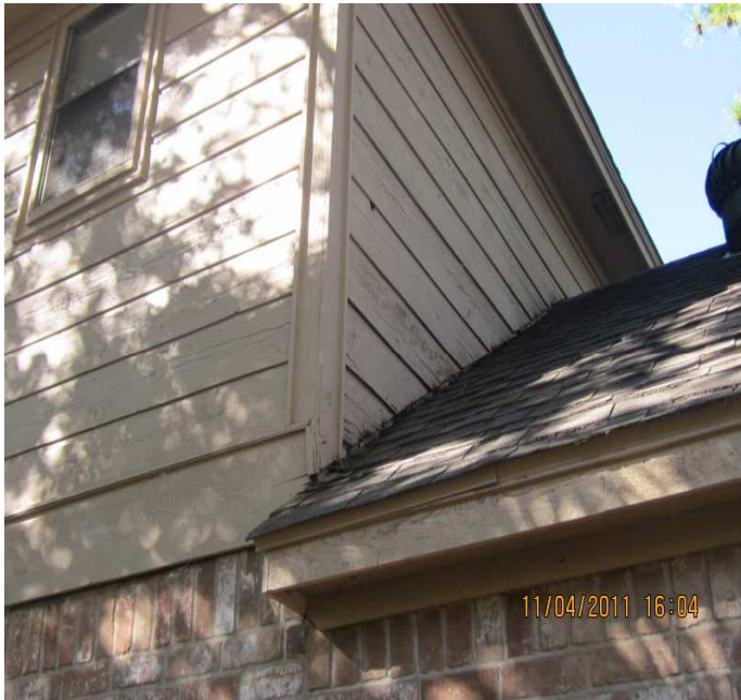
PHOTO NO. 11 DAMAGED EXTERIOR SIDING UPPER BACK EAST SIDE
