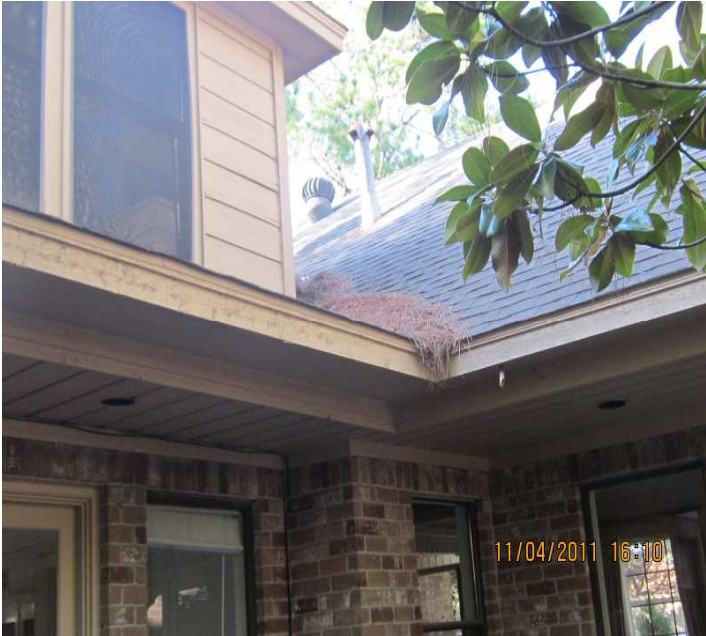
PHOTO NO. 15 PINE NEEDLES IN ROOF VALLEYS
