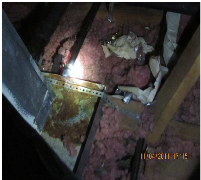
PHOTO NO. 28 A/C DRAIN PAN FULL OF RUST & MISSING FLOAT SWITCH
