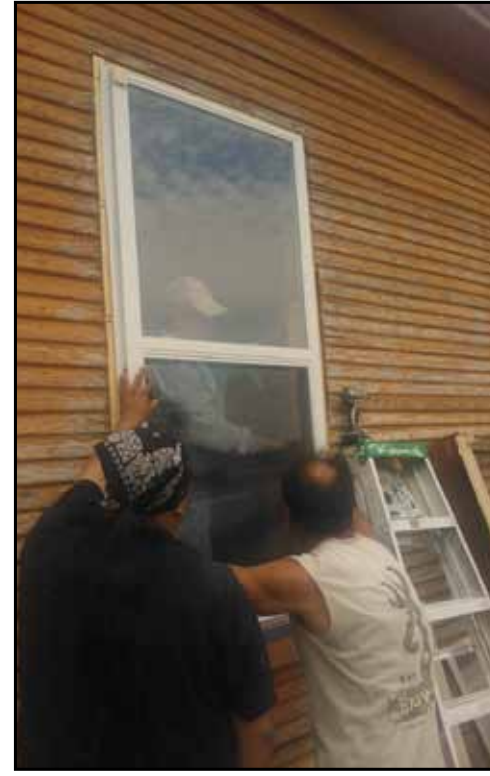
Dusty Eaves (left), Ronnie Cooper (right) and Sonny (Arthur) Fields (inside) install and seal the new, double-glass windows.
