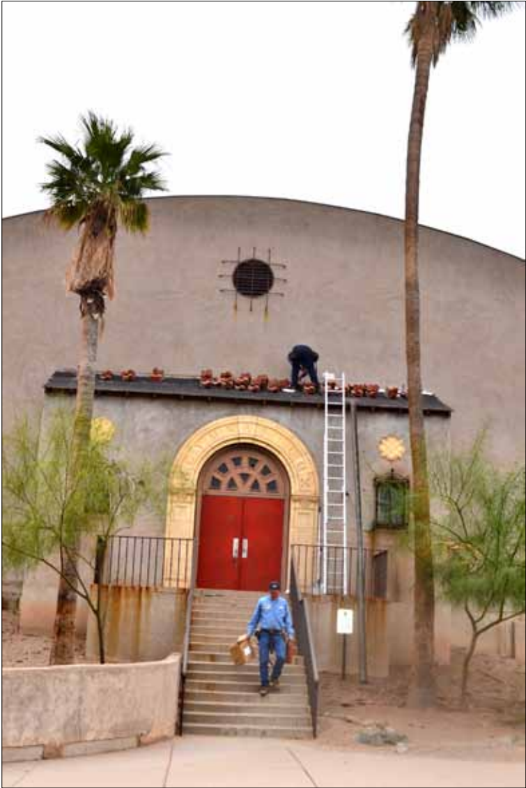
The historic Curley School gymnasium is undergoing some needed repairs. The county has subcontracted work to replace roof tile, and repair the exterior wall on the west of the building to protect it from further water damage. “The work being done is to stabilize the structure and prevent further erosion of the building,” said Terry Leatherwood of Pima County Natural Resources Parks & Recreation.
