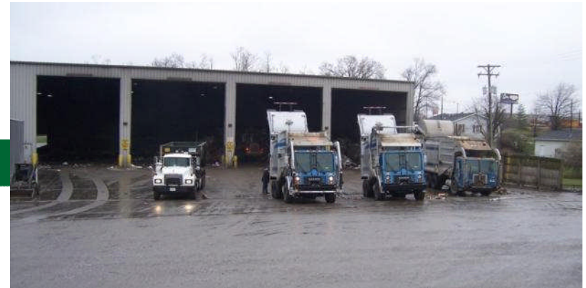
↑ Construction of Commercial Transfer Station for Waste Export
