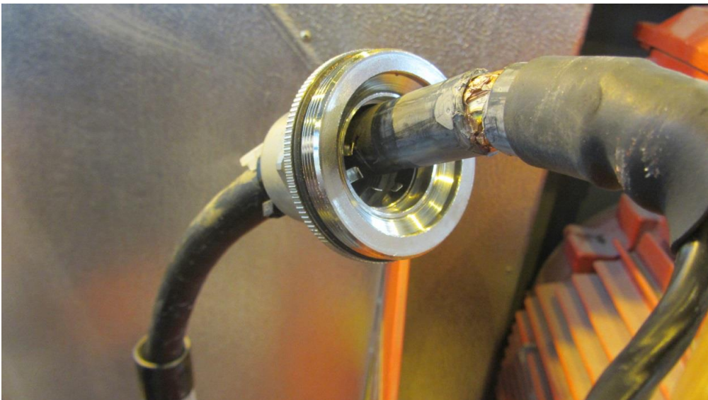
Figure 28. An EMC cable gland is used for connecting the supply cable to the cable terminal box. Many of the connection pins to the cable screen were broken at the 1HTC20AN001 (Bag filter preheating fan) motor. This gland was replaced.
