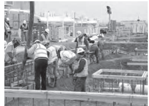
Workers are constructing an Annex that will support the sludge retrieval and transfer equipment at the K-West Reactor.
