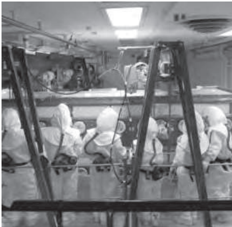
Workers in full protective and respiratory equipment install hoisting connections prior to initiating the lift to separate a 10-ton glovebox at the Plutonium Finishing Plant.
