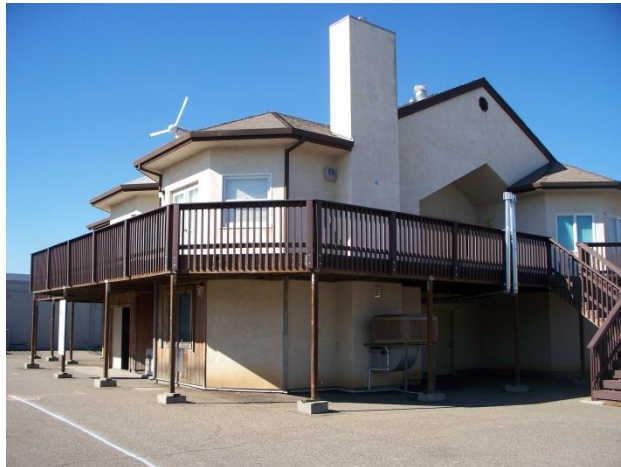
FIGURE 3. EXISTING "HOME" FACILITY AT STOCKTON ETC
