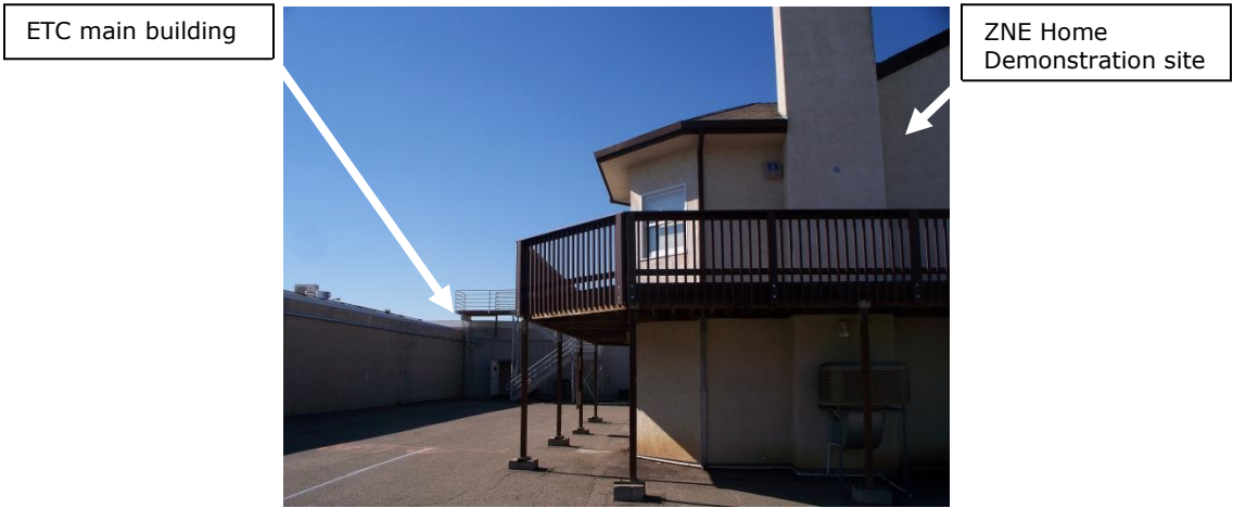
FIGURE 4. LOCATION OF "HOME" FACILITY (ON RIGHT) RELATIVE TO MAIN ETC BUILDING (GRAY BUILDING ON THE LEFT AND IN THE BACKGROUND)
