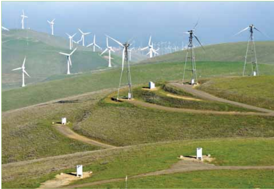
Repowering will replace older, poorly located wind turbines with less than one-tenth as many larger, more efficient and micro-sited turbines, hopefully decreasing terrestrial impacts and on birds and bats.
