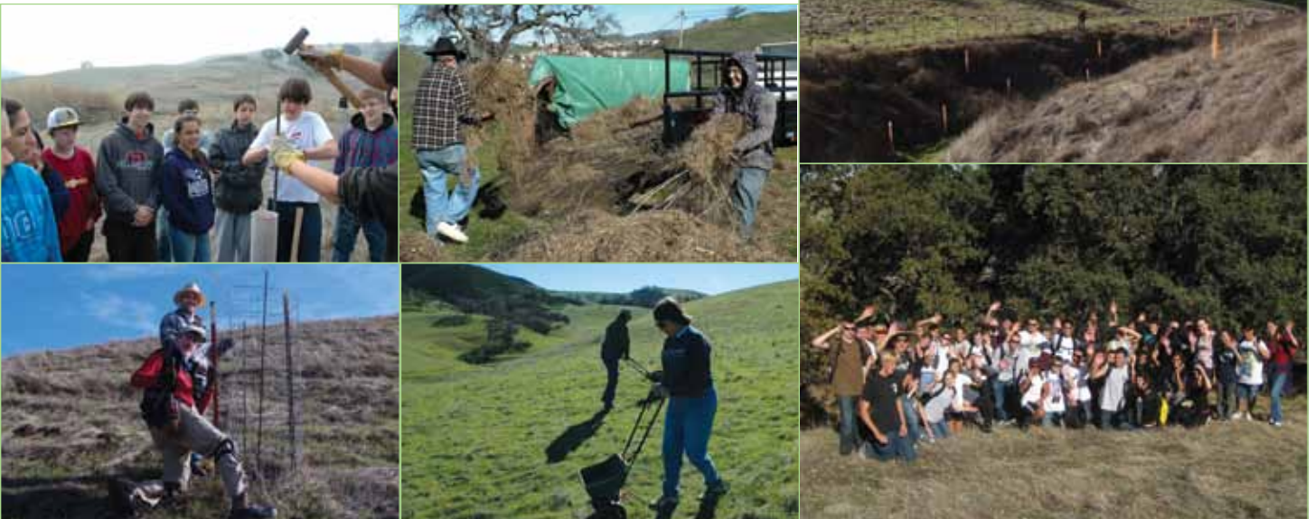
(clockwise) Northgate High students learn to install plant tubes; Dave Sargent and George Phillips load the trailer; Plant tubes protect oaks and buckeyes at Irish Canyon; Northgate students learn about restoration; Kristen Wick and Bob Busch spread seeds on a hillside; Brad Heckman and George Phillips protect trees from cattle.
