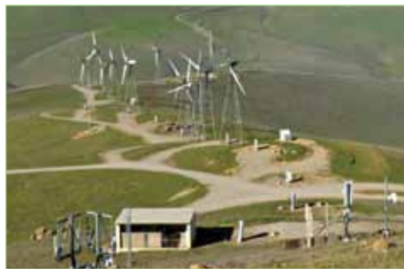
Every wind turbine is served by an individual, erosion-prone maintenance road. Fewer turbines equals fewer roads and less terrestrial impact.
