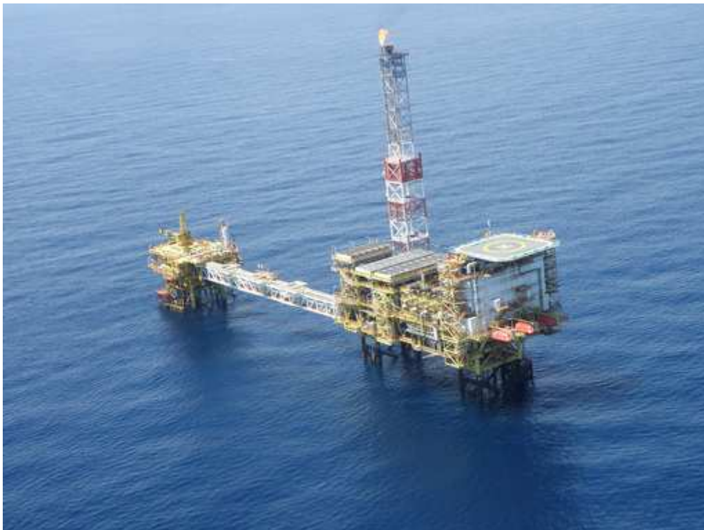
Figure 1: an offshore helideck (Helideckinspect, 2013)
