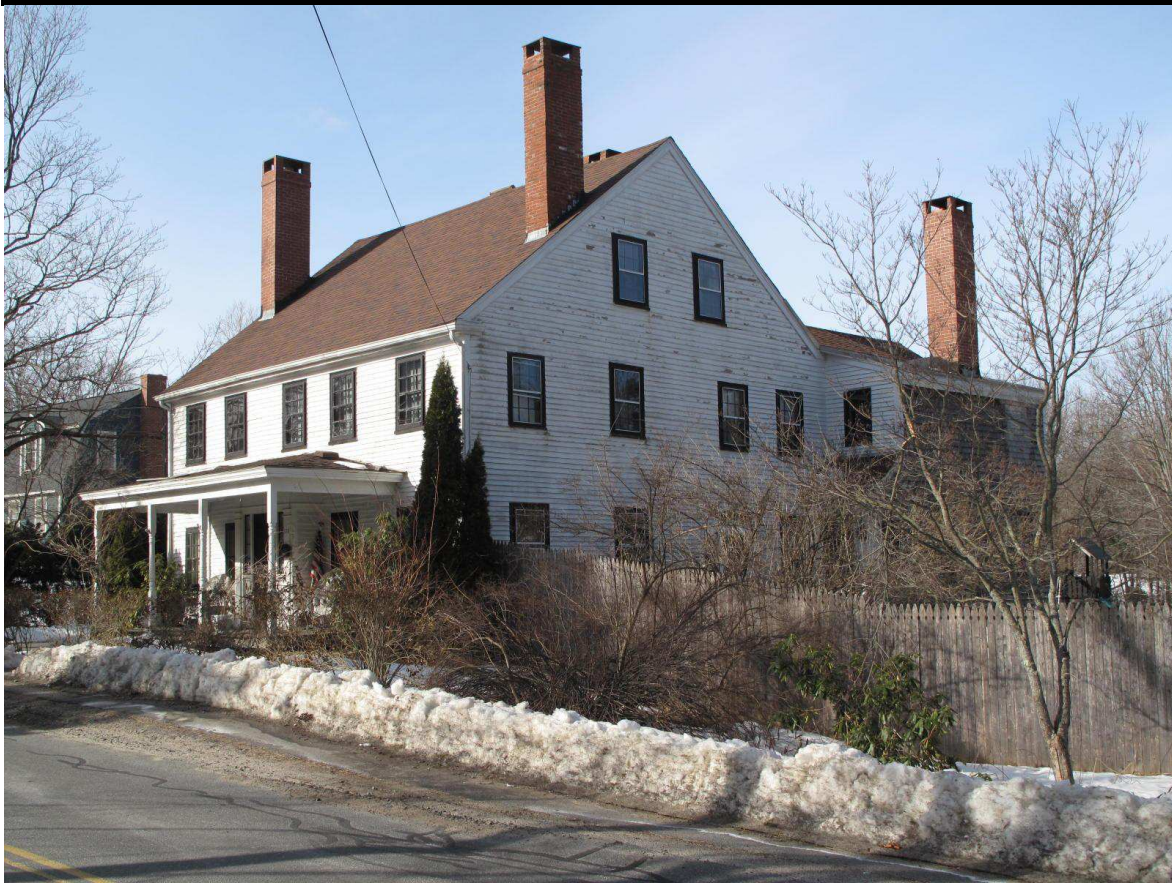
View from NE
