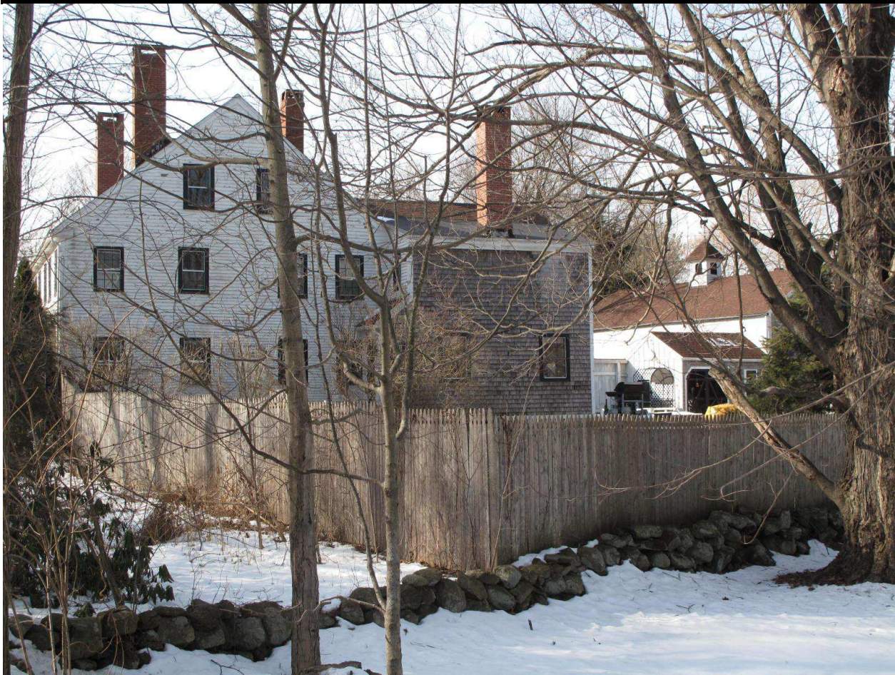
View from NE
