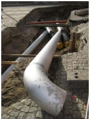
Unprotected type 304L drinking water pipe in the city centre of the Swedish capital Stockholm.
