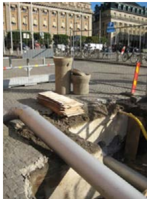
Unprotected type 304L drinking water pipe in the city centre of the Swedish capital Stockholm.
