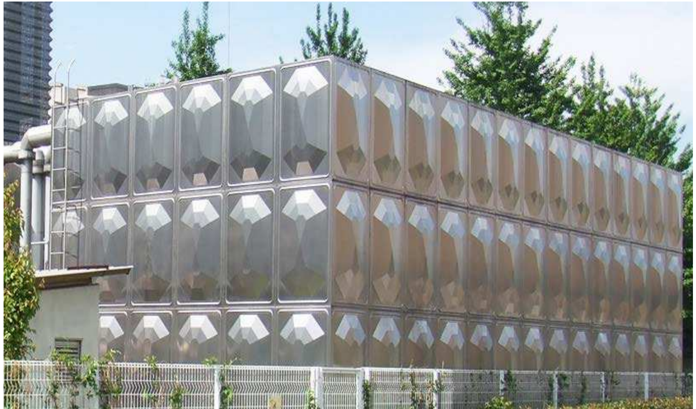
Modular water tank system made from stiffened stainless steel panels. Photo: Morimatsu (Japan), www.morimatsu.co.jp
