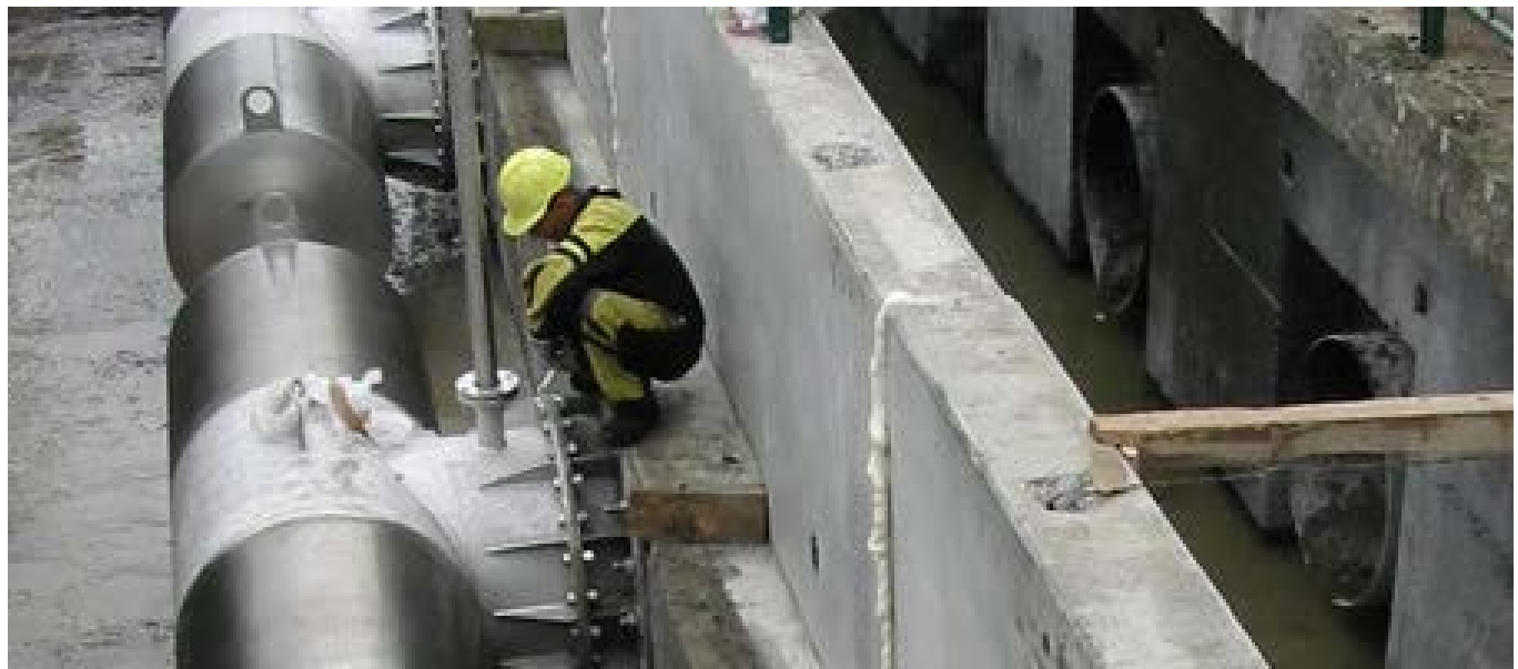
Intake for river beds. Source: Euroslot Kdss (UK), www.euroslotkdss.com
