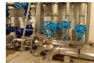
Stainless steel in a typical mixed-material installation can be combined with coated steel and cast iron parts provided the connections are properly designed and the flow direction is taken into account.
