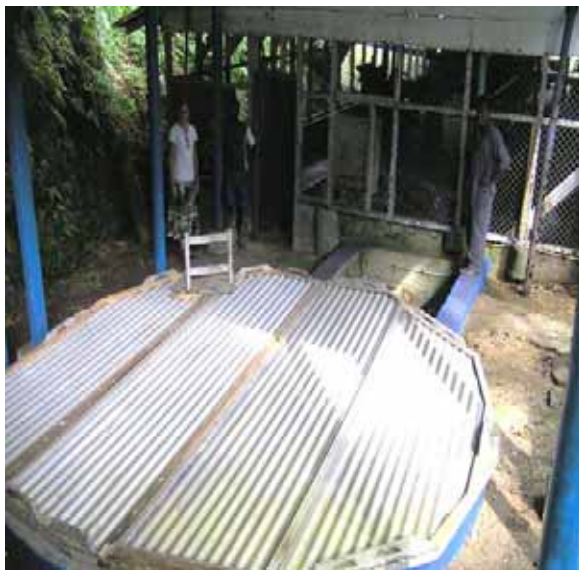
Luganville water supply intake well
