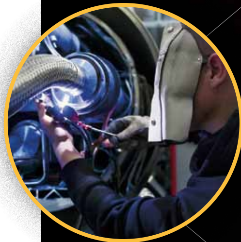
Welding one of the final LHC interconnections. A welder works on the interconnection between two of the LHC's superconducting magnet systems, in the LHC tunnel.
