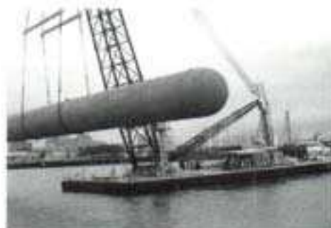
Harbor Service/Derrick Barge
