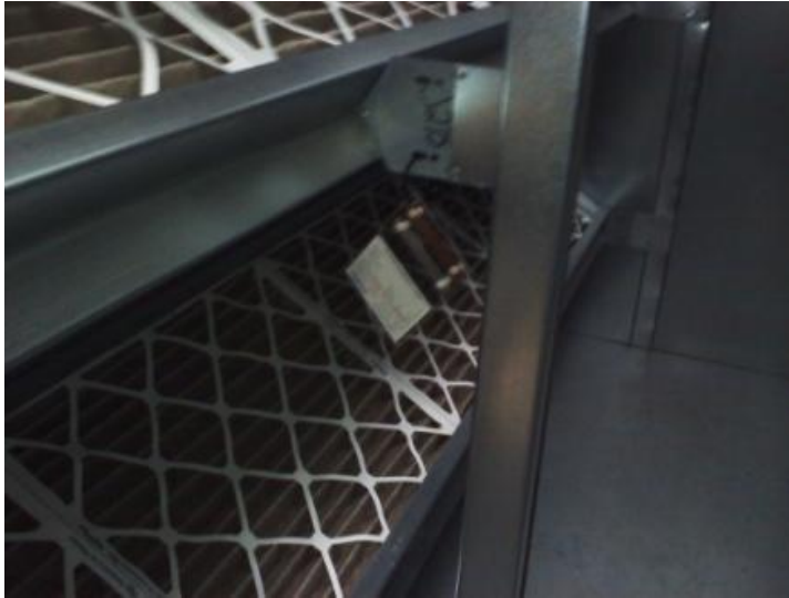
Figure 4 - Typical Coupon Mounting - Example Shown at Supply Air Filters as Found in Large Roof Top Fan Units
