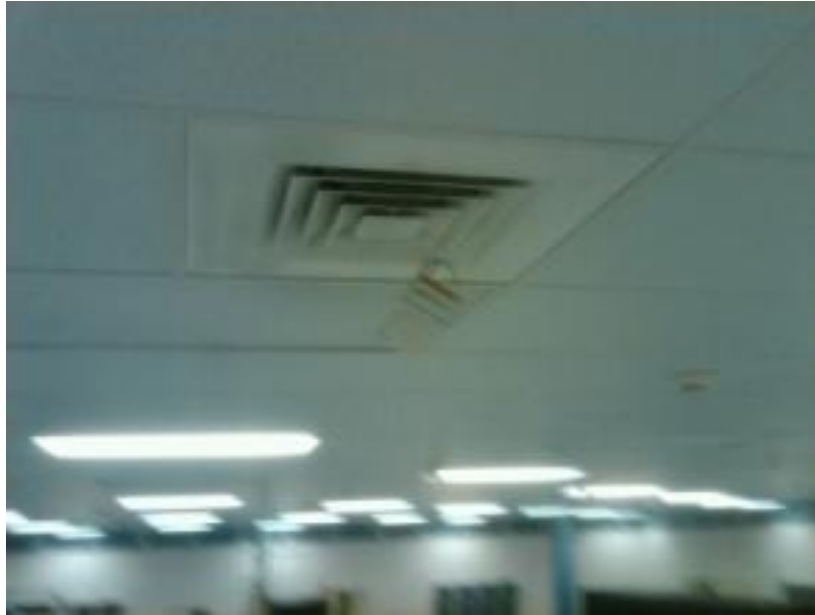
Figure 6: Typical Coupon Mounting, Example Shown at Data Center Room Supply or Return Grill
