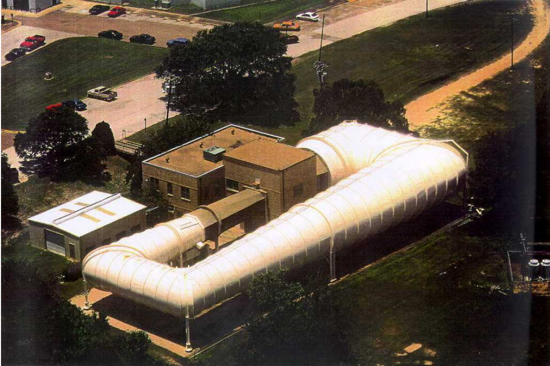
Figure 2. Aerial photograph of the Oran W. Nicks Low Speed Wind Tunnel Facility.
