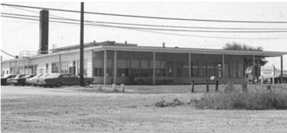
In 1967 this building served as the Technical Center for the WCC Willow Run campus.
