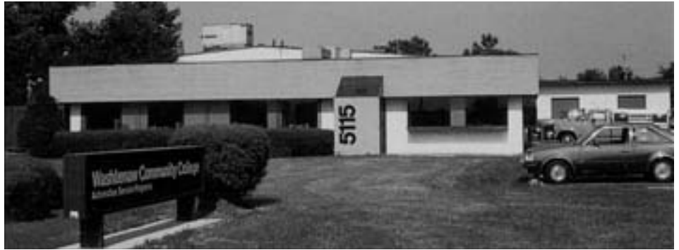
WCC also purchased the former dairy distribution center on Carpenter Road to house the Automotive Services Program. Top photo shows facility in 1966 and bottom photo shows facility in 1979 following renovation and expansion.
